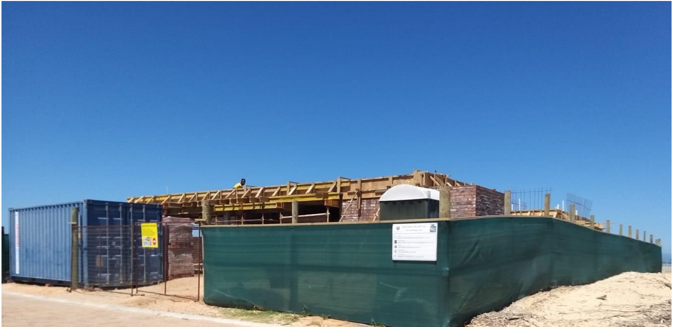
Photo 3: The first floor deck of the house being built on Erf 2421 has been prepared for casting the concrete. The site has a toilet and a skip on site for builder's rubble. The chemical toilet is also visible on site. The site was in a neat and tidy condition.
