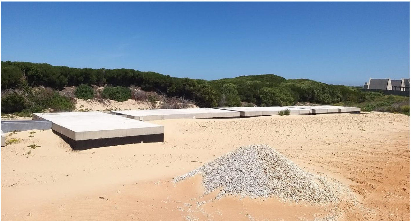
Photo 6: The final lids have been placed onto the various tanks of the package sewage plant.
