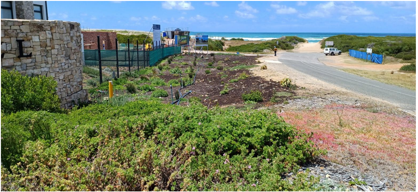
Photo 7: The Preekstoel road reserve has been cleared of alien vegetation and has been landscaped with Blombos Strandveld species. A temporary irrigation system has been placed on the surface of the landscaped area.
