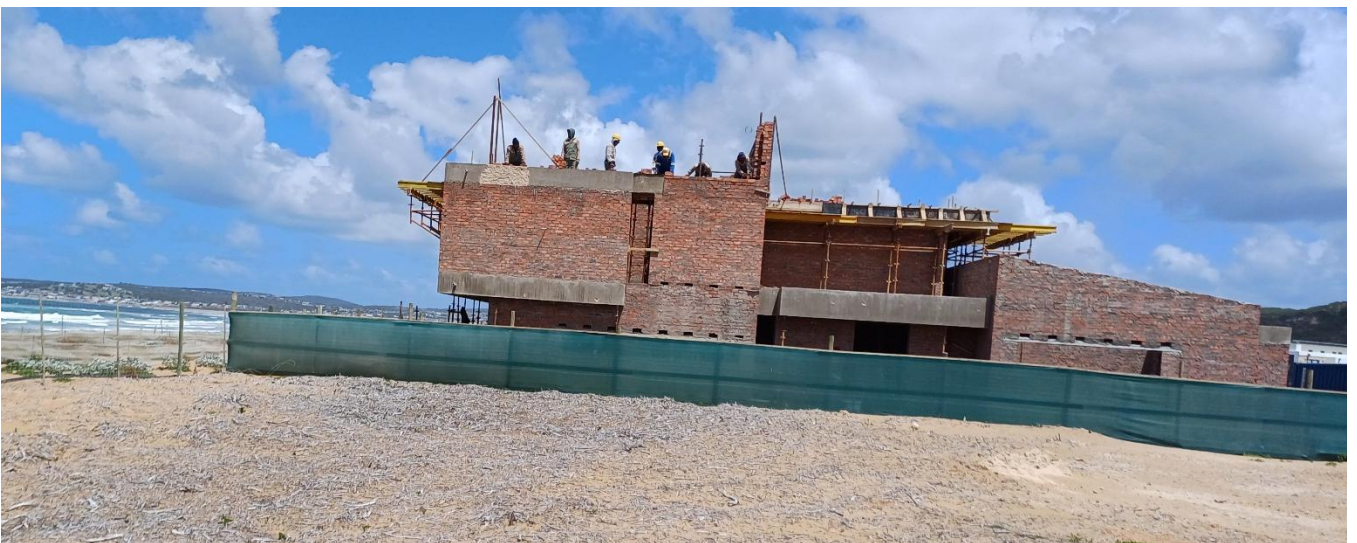
Photo 3: The first floor of the house being built on Erf 2421 was nearing completion on 5 March 2025.
