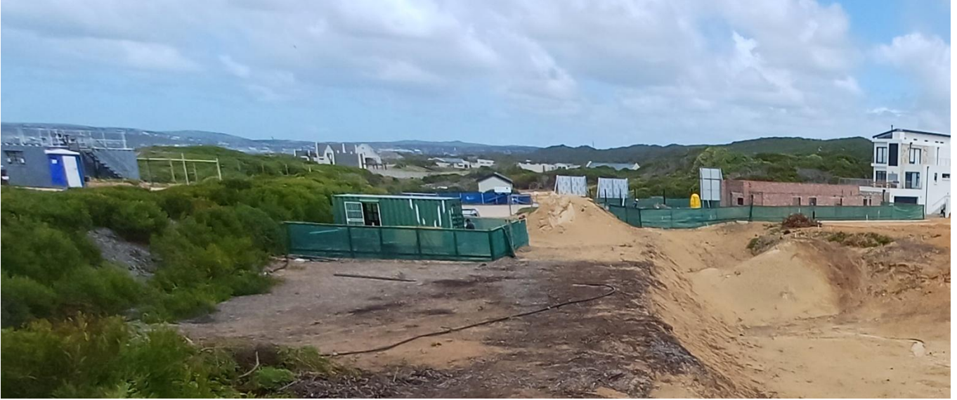
Photo 1: The Chel Building & Civils yard and the building site of Erf 2458 were in a neat and tidy state.
