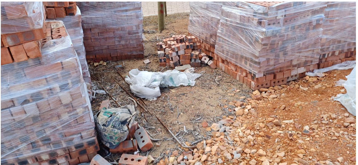
Photo 4: The contractors were reminded to pick up the plastic wrapping from the bricks and place in dust bins.
