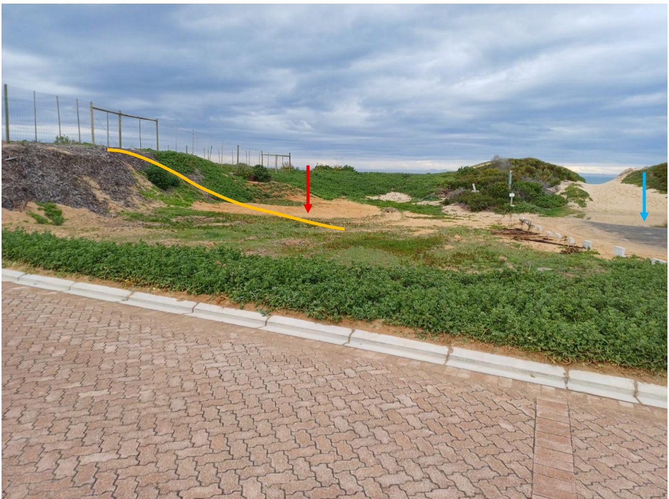
Photo 7b: The Provincial Road Reserve is from the western fence to the edge of the Preekstoel road. The red arrow shows where the deep erosion area of the lee side of the frontal dune has been filled with sand. The recommendation is to place sand fill between the terrace within Preekstoel Beach Estate and gently slope it towards the road. This area will then be landscaped with Blombos Strandveld plant species. Note the accumulation of stormwater at the foot of the dune (blue arrow). The old access road to the hotel site will be removed and landscaped.
