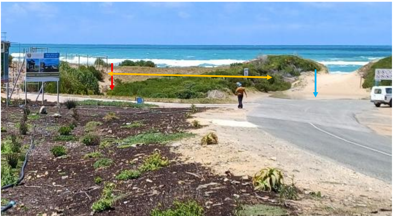
Photo 7a: The Provincial Road Reserve is depicted by the orange double-headed arrow. The mainly invasive, exotic rooikrans shrubs have now been removed (refer to Photo 7b). The blue arrow shows the accumulation of stormwater and the red arrow shows the deep erosion area in the lee side of the frontal dune.
