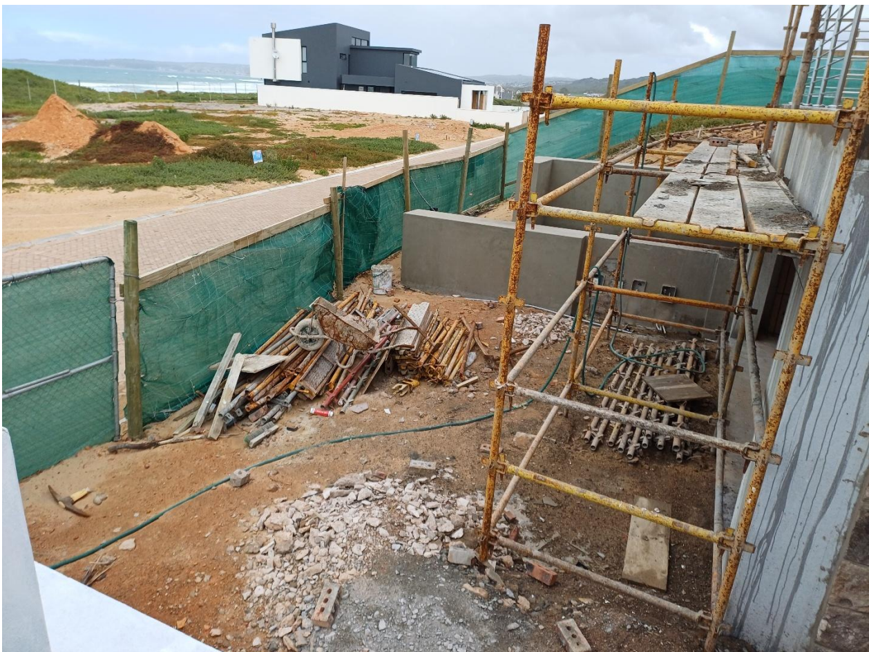
Photo 4: Builder's rubble, planks, a broken pick and scaffolding lying around one of Woudt Building's sites.
