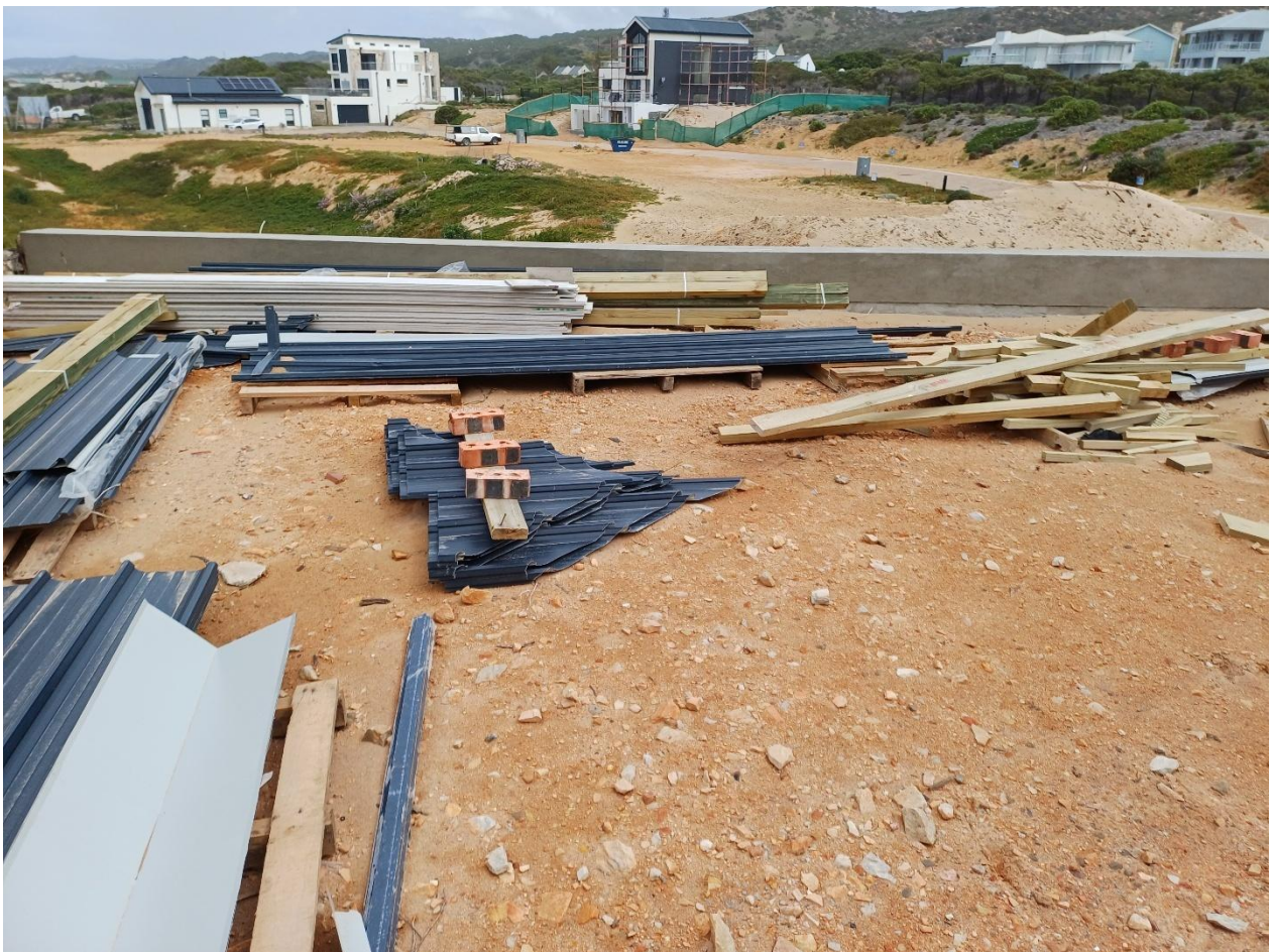
Photo 5: Whilst the metal roof sheeting is reasonably neatly stacked on site, cut-off roofing timber and bricks litter the site.
