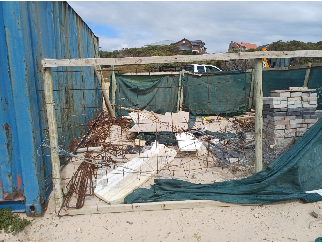
Photo 2: Hap-hazard storage of building materials in the Woudt Building site yard.
