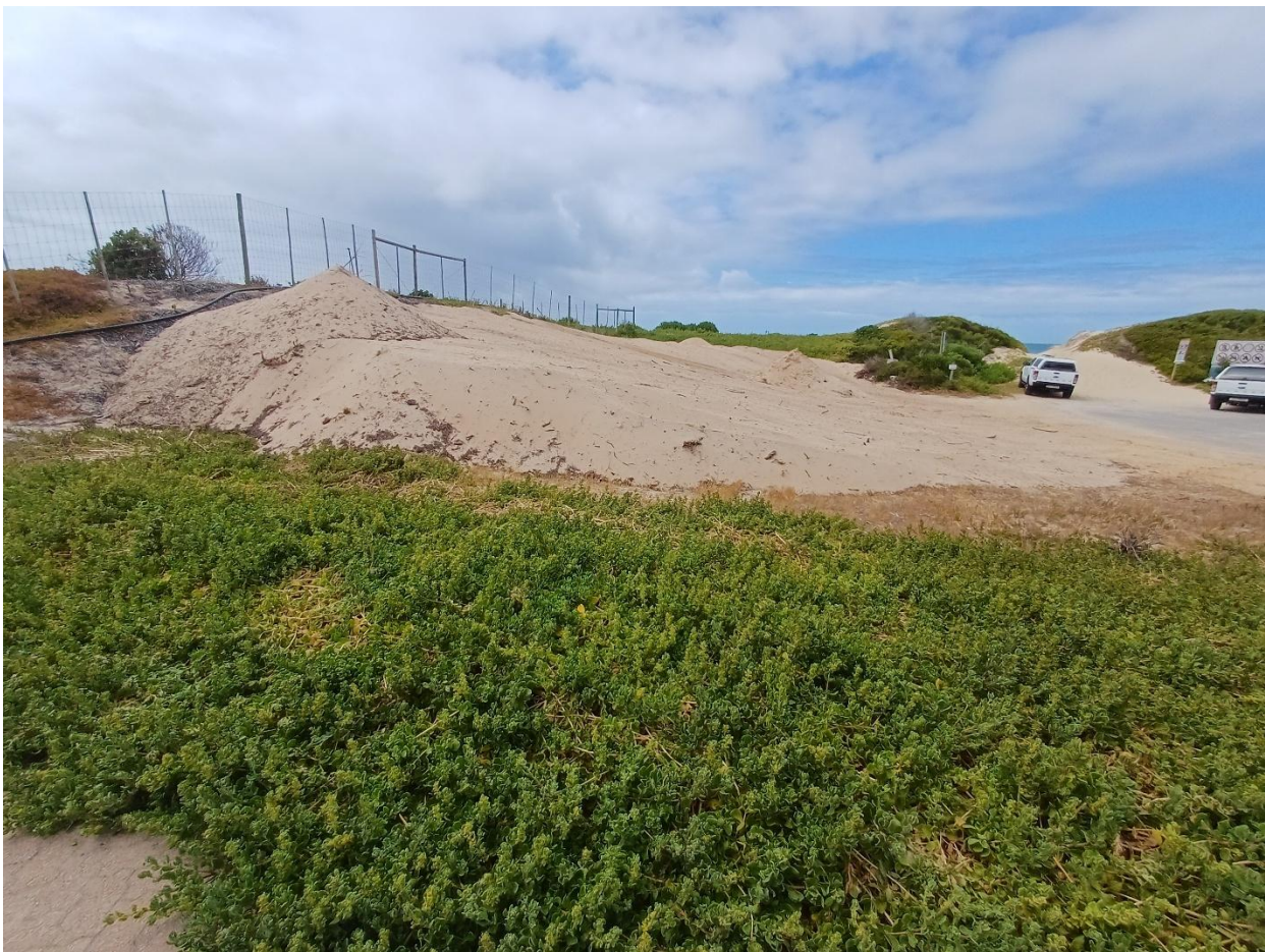
Photo 13: The section of the road reserve at the end of the Preekstoel road has been filled with sand and will be landscaped with pioneer Cape seashore creepers and Blombos Strandveld plants species.
