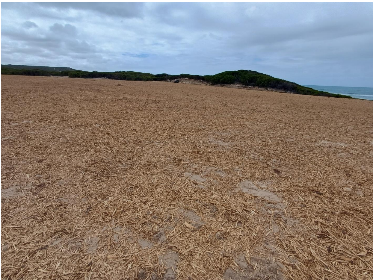
Photo 7: The building platform for Phase F has been completed and covered in wood chips to prevent wind erosion. The installation of roads, sewage pipes, stormwater, water and electrical reticulation will start in January 2026.
