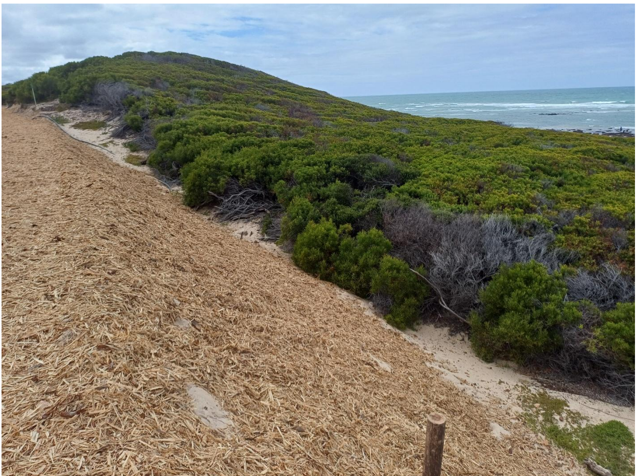
Photo 8: The southern edge of the stabilized building platform of Phase F has been completed. This sloped edge will be landscaped with Blombos Strandveld plants and Cape Seashore creepers.
