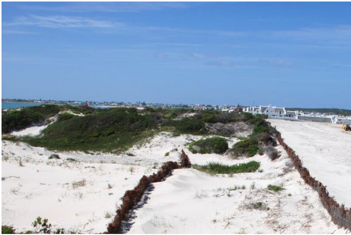
Photo 7: A: Shows two brushwood fences that were constructed across a large blow-out structure within the frontal dune system in the Langezand Phase 2 project (Struisbaai) area to trap sand. B: Shows the same area, three months later. Note how much sand was trapped by both brushwood fences. The aim here was to recreate a stable back-dune across the blow-out as shown by the yellow lines. Once sufficient sand has been accumulated, the dune would be planted with locally indigenous strand plants (pioneers) and more climax strandveld plants.
