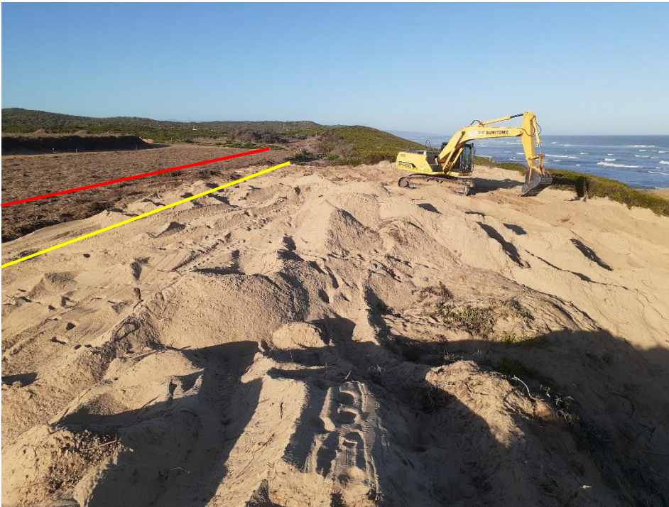
Photo 8: Shows the movement of sand from the back dune area towards the hummocky dunes just above the spring tide mark with an excavator. The stable platform for the construction of houses is seen to the left of the photo, which has been covered with chipped rooikrans mulch. The yellow line represents the conservation setback line or ecological setback line that was determined for the development. The area between the yellow line and the high water mark represents Erf 2341. The red line represents the 5m building line.
