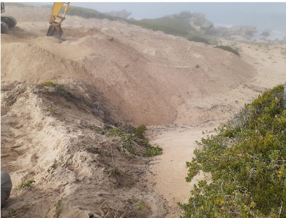
Photo 11: Shows the filling in of large blow-outs with sand moved from the back dune area. Most of the remnant dune system had originally been stabilised by planting rooikrans in the early 1900's (8 August 2022).
