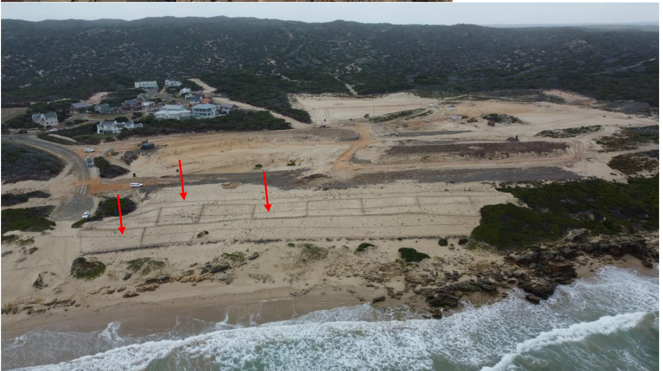
Photo 14: A drone photo of the rehabilitated dune system showing the erosion prevention netting in place and the temporary irrigation system (red arrows). Note the hummocky dunes (photo taken on 10 November 2022).
