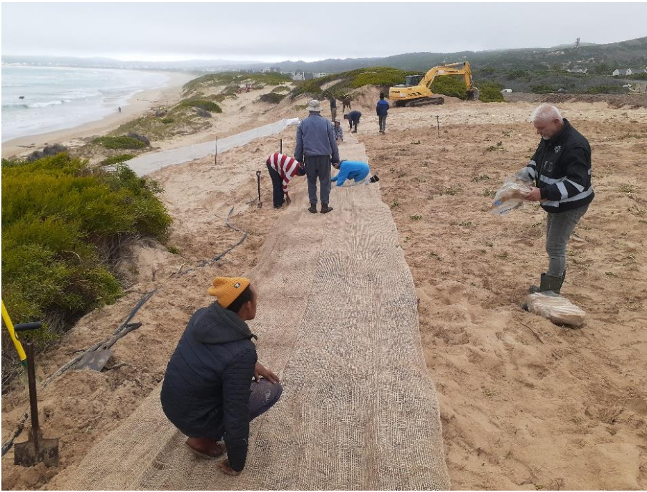
Photo 12: Once all the back dune sand had been moved to the hummocky dunes, shade netting was erected near the hummock dunes. A “soil-saver” hessian blanket was pegged to the sand at the apex of the slope of the frontal dune system to prevent erosion (10 August 2022). Deon van Eeden is seen to the right of the photo, supervising the specialist rehabilitation team from Still Bay.
