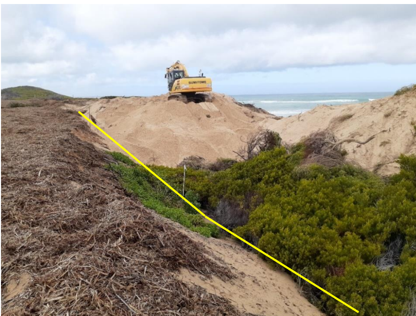
Photo 9: Shows the movement of sand from the back dune area by excavator. Note the steep angle of repose of the dune to the right which is caused by the rooikrans vegetation that holds the sand as it cascades over the back of the dune caused by wind erosion from blow-outs. Note the stabilised building platform covered in mulch from the chipping of rooikrans removed from the development area. The wooden stakes at the edge of the building platform is the alignment of the conservation setback line (8 August 2022). The area between the stabilised platform and the dune to the right was filled in with sand removed from the back area of Erf 2343.
