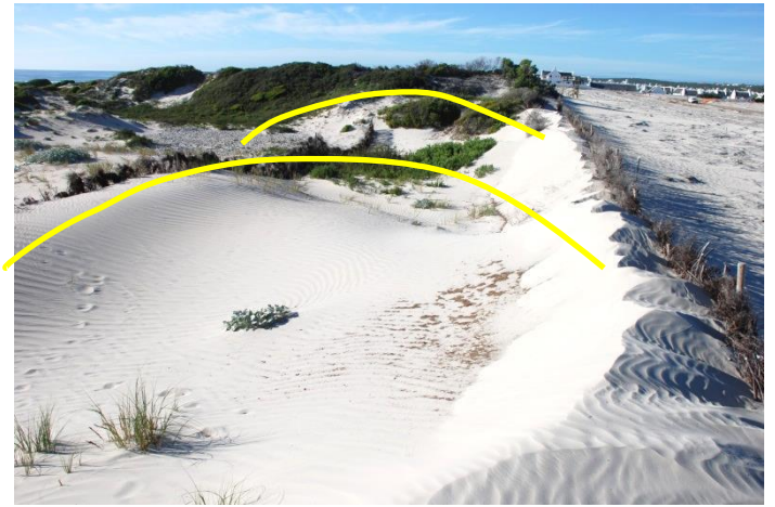
Photo 7: A: Shows two brushwood fences that were constructed across a large blow-out structure within the frontal dune system in the Langezand Phase 2 project (Struisbaai) area to trap sand. B: Shows the same area, three months later. Note how much sand was trapped by both brushwood fences. The aim here was to recreate a stable back-dune across the blow-out as shown by the yellow lines. Once sufficient sand has been accumulated, the dune would be planted with locally indigenous strand plants (pioneers) and more climax strandveld plants.
