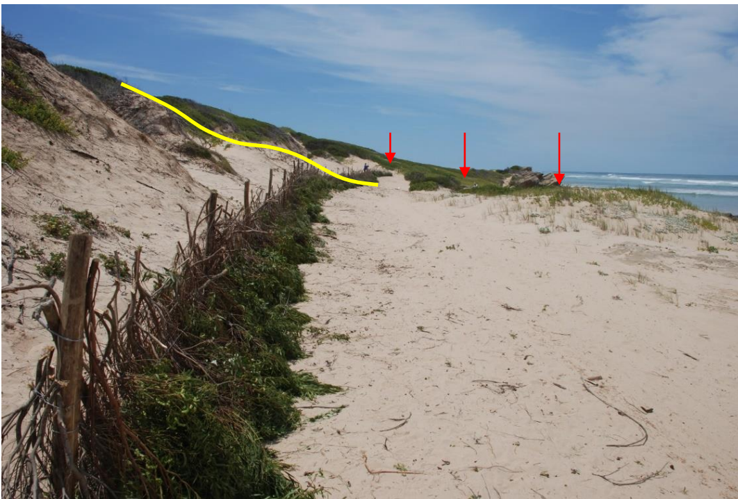
Photo 6: This photo was taken of the frontal dunes at Preekstoel where a brushwood fence was erected in front of the dunes just landward of the hummocky dunes (red arrows). The brushwood comprises rooikrans bushes that have been removed from the backdune system to be woven between the horizontal strands of wire. The idea was that the brushwood fences would trap sufficient sand (yellow line) so that the front of the dune could be rehabilitated by planting climax Strandveld plants and various hardy pioneer strand plants ( Photo 6 was taken on 5 November 2021).
