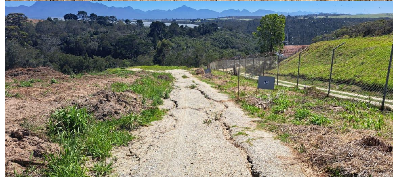
Image 10: Erosion observed on sloping single track road.
