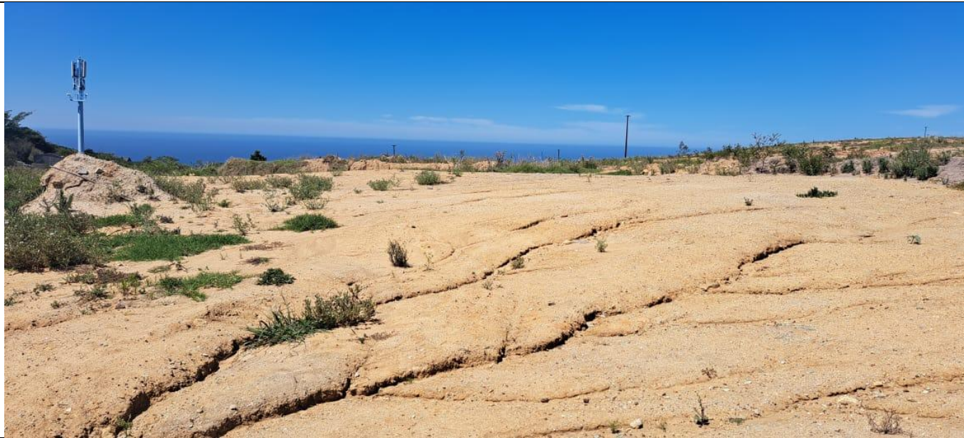
Image 13: Erosion observed on exposed slopes and roads. Runoff causing rills and formation of gullies (potential gully erosion).
