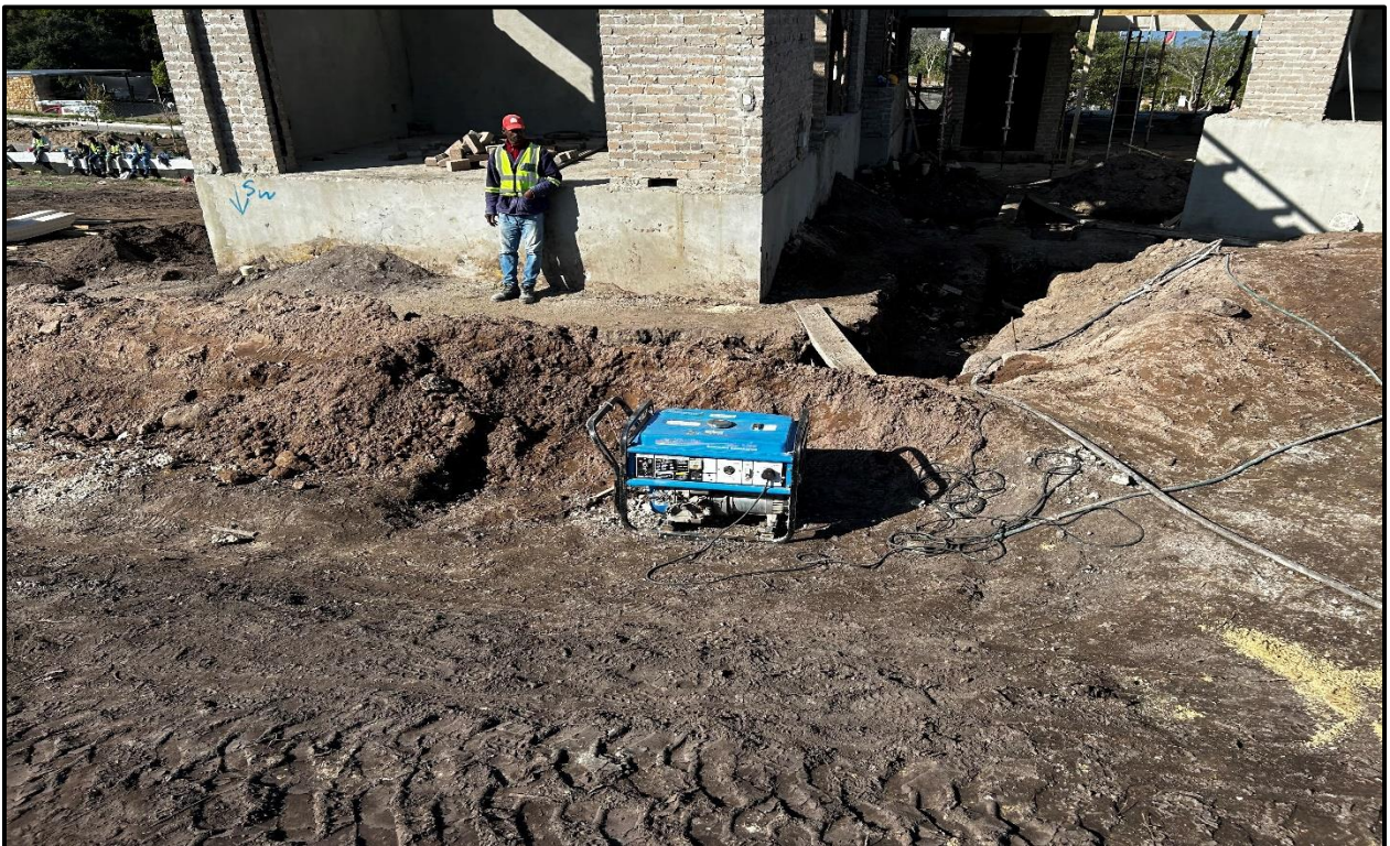
Image 4: Generator not on drip tray (26/06/2024).
