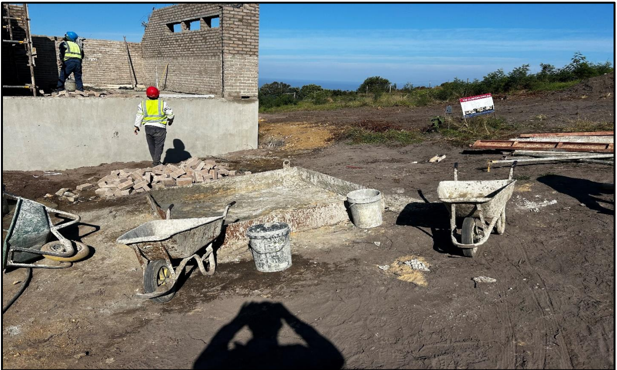
Image 4: Concrete batching on boards.
