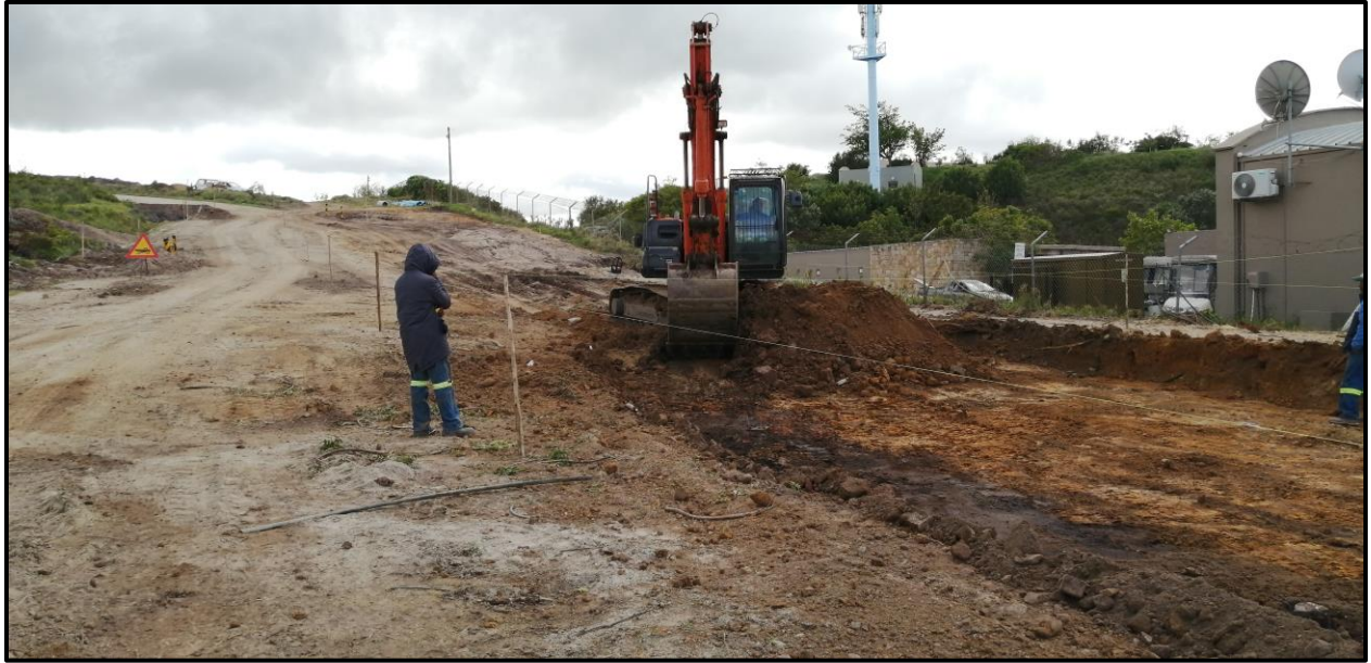
Image 3: Soil excavation for road construction
