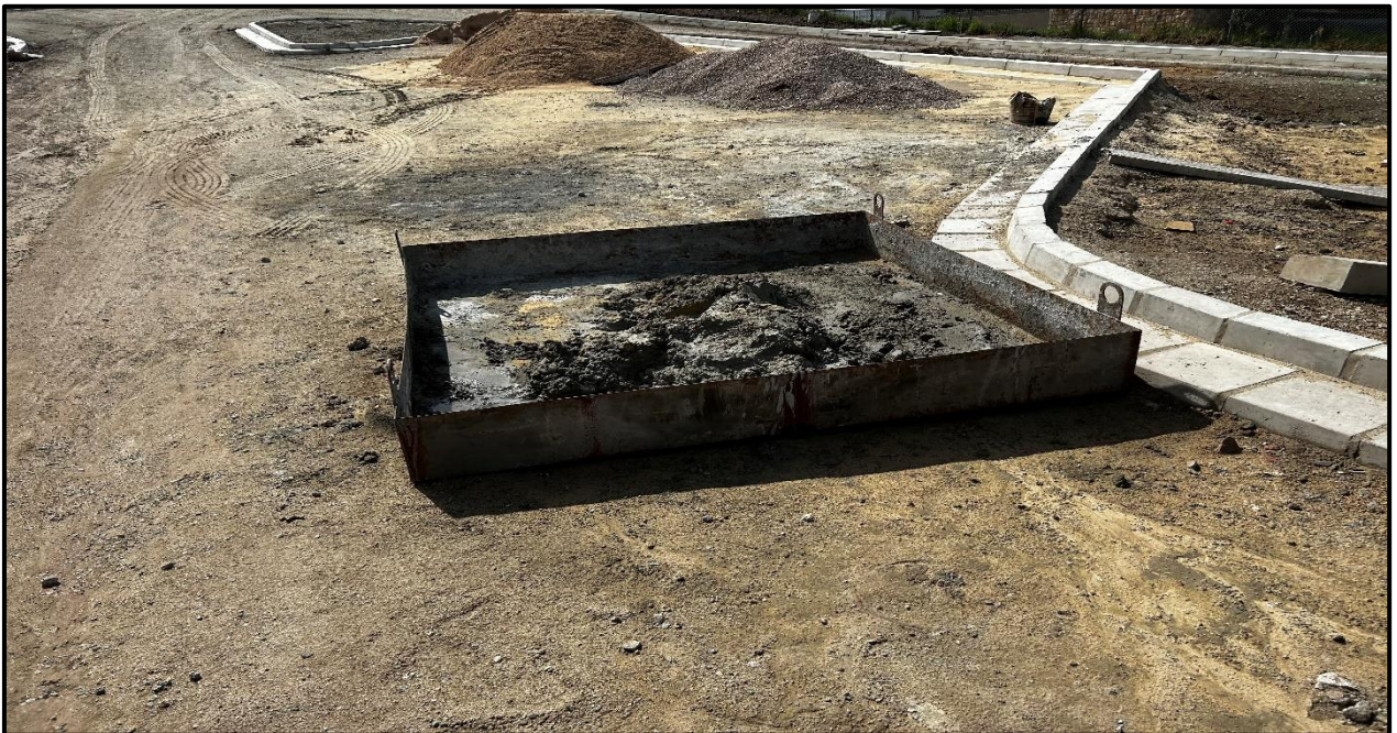
Image 6: Concrete mixing on boards.
