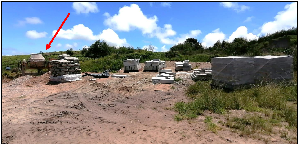
Figure 4: Construction material on site and cement/concrete mixer that must be on an impermeable/bunded surface.
