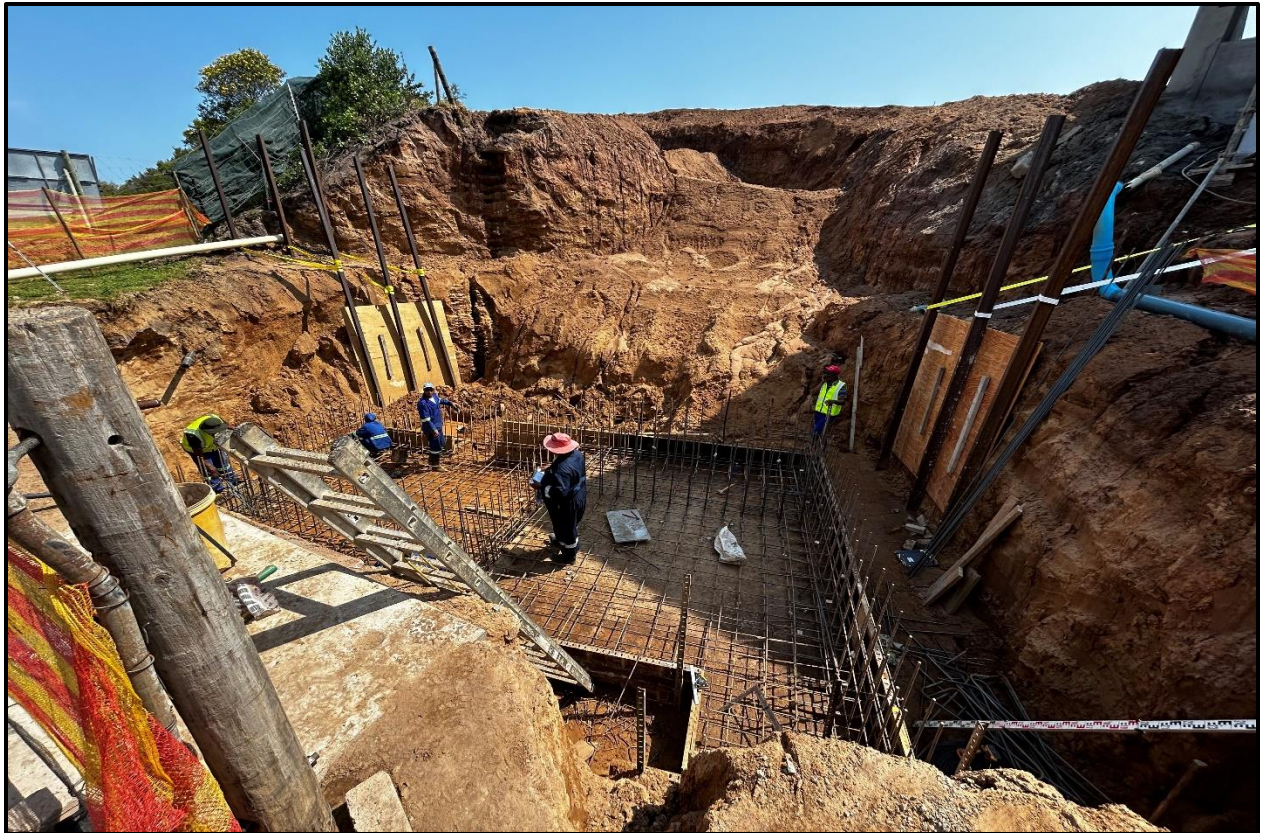
Image 1: Construction of sewage package plant.
