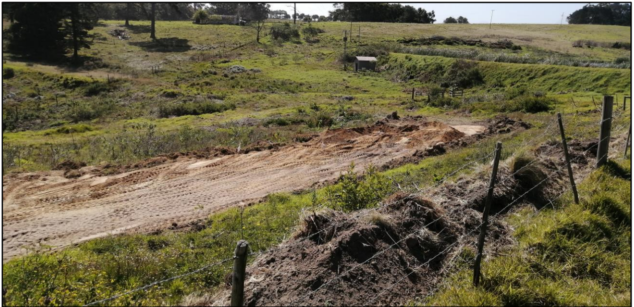
Image 6: Soil excavated and vegetation cleared for road construction.
