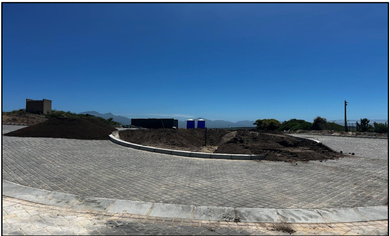
Image 3: Construction of traffic circle.
