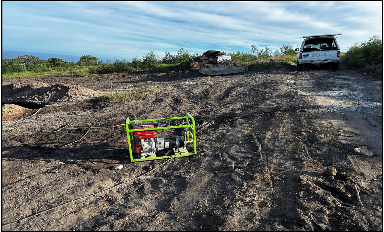
Image 5: Generator not on drip tray and concrete spillage (20 June 2024).
