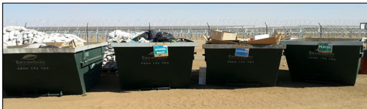
Figure 4: Recycling system implemented on a construction site. Skips provided for general waste, plastic, cardboard and metal.
