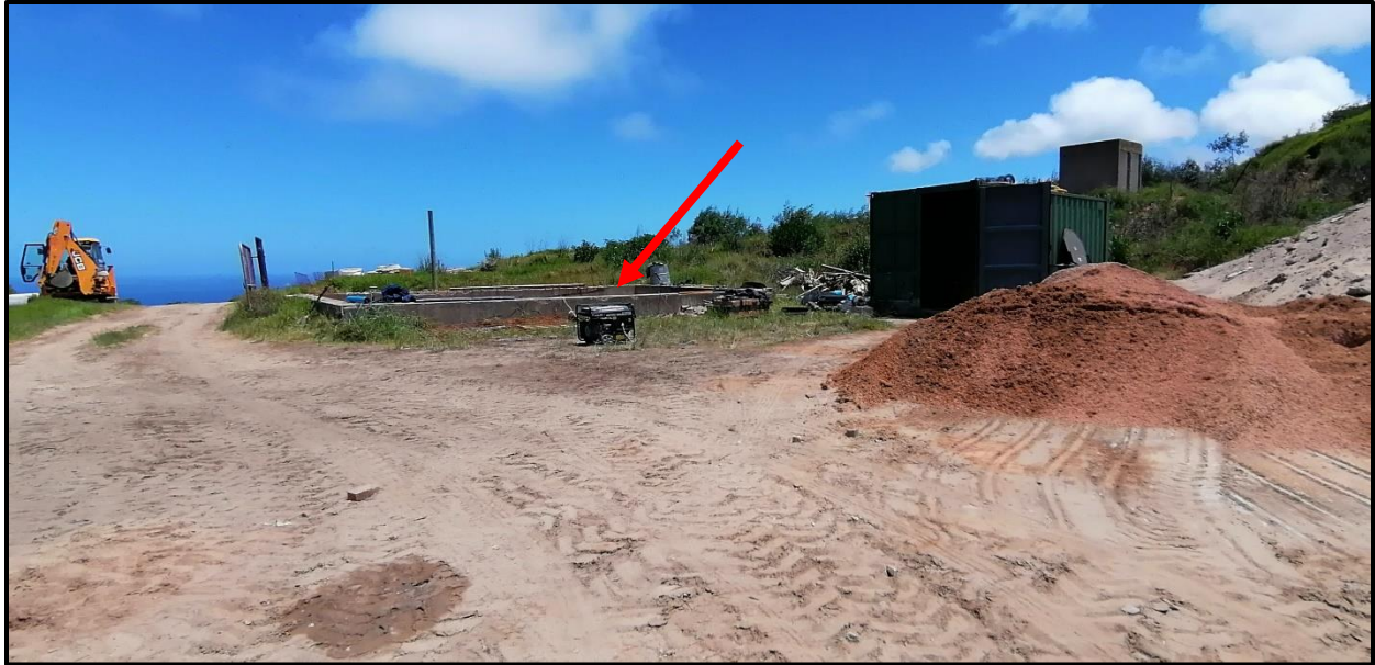
Image 5: Generator that needs to be on a drip tray.
