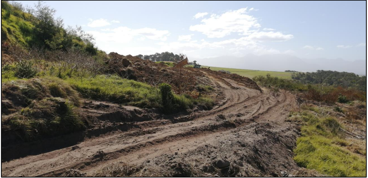
Image 5: Soil excavated, and vegetation cleared for road construction.
