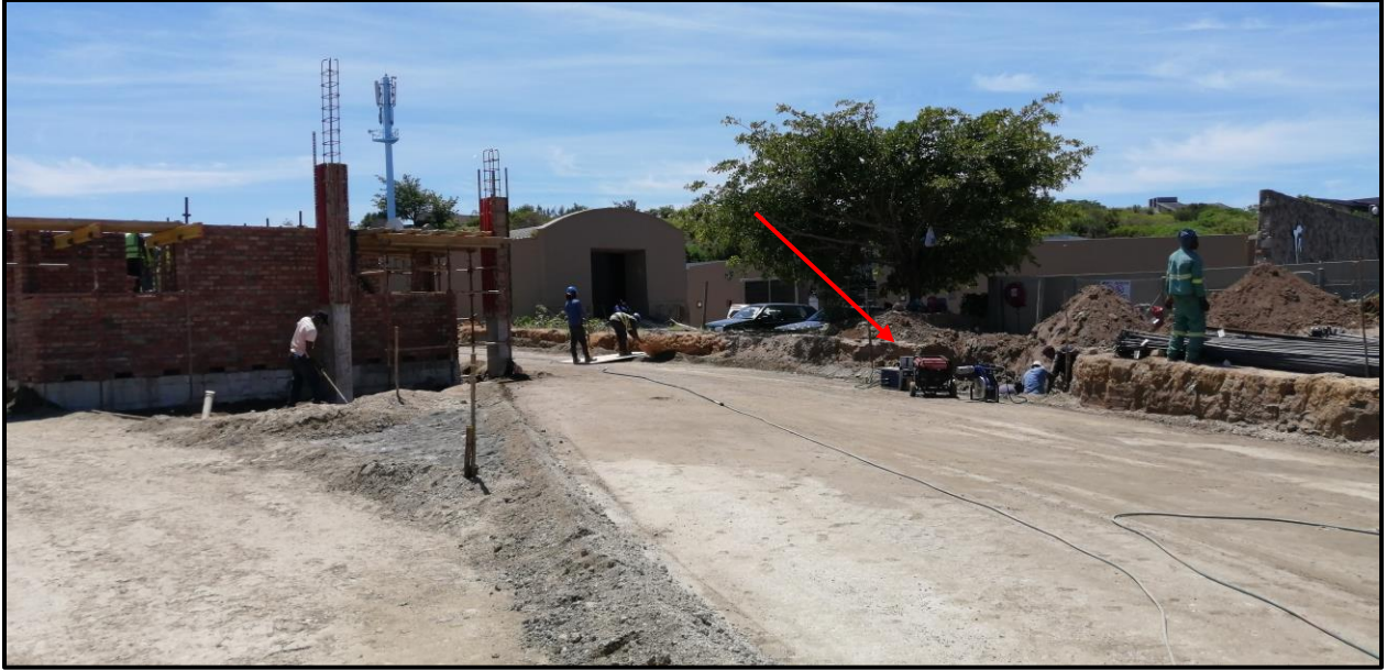
Image 17: Generator that must be on a drip tray.
