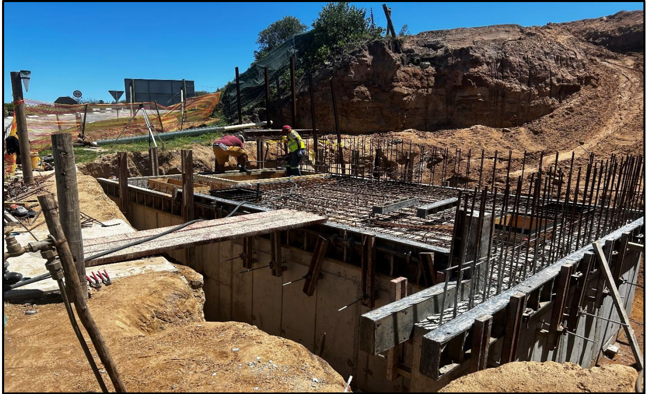
Image 2: Construction of sewage package plant.
