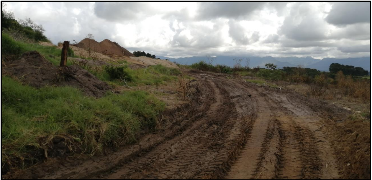
Image 8: Excavated soil and vegetation clearance for road.
