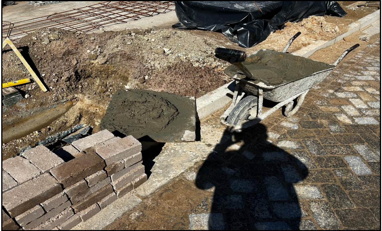
Image 7: Concrete batching on boards.
