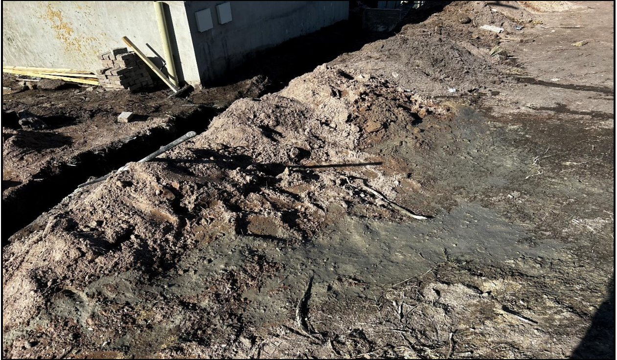
Image 3: Concrete spillage on site (26/06/2024).
