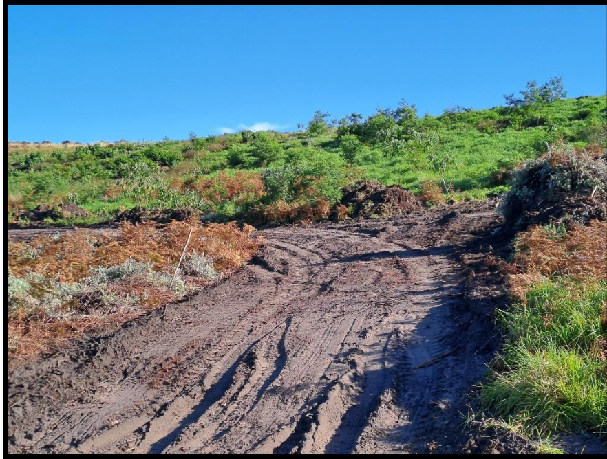
Image 2: Soil excavated and vegetation cleared for road construction.
