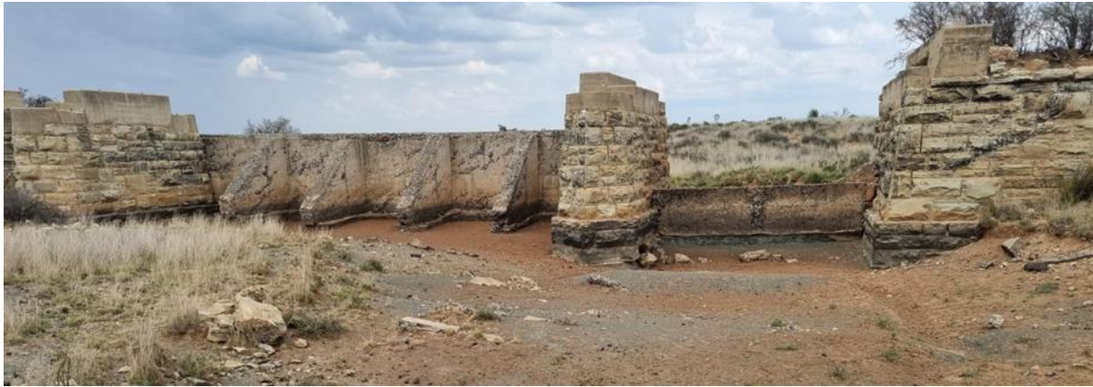
Figure 3-12: Instream dam with associated weir along the Brak River
