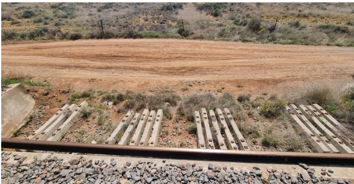
Figure 3-14: Railway crossing the tributaries of the Roodekraal River
