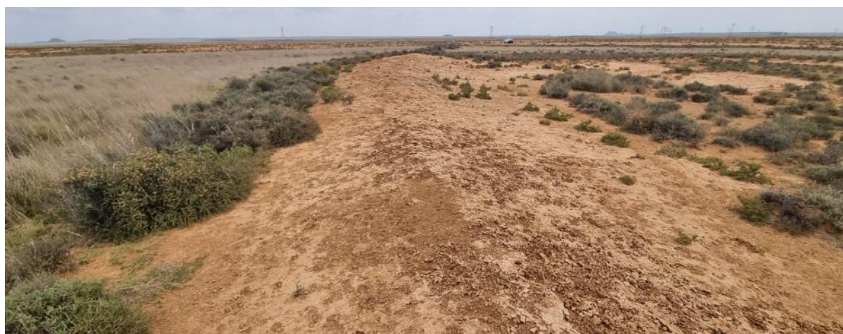
Figure 3-11: Dam wall at BR T1
