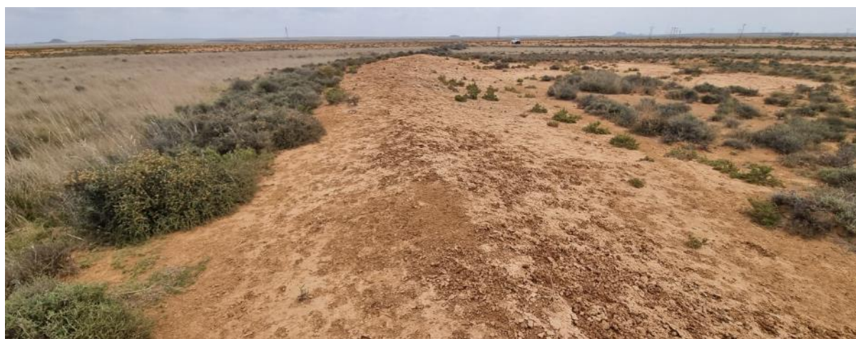
Figure 3-11: Dam wall at BR T1
