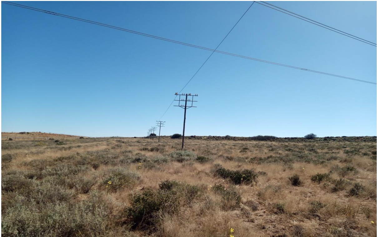
Figure 48: remnant telephone infrastructure
