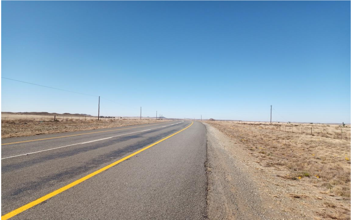
Figure 36: View from the N10 looking southeast
