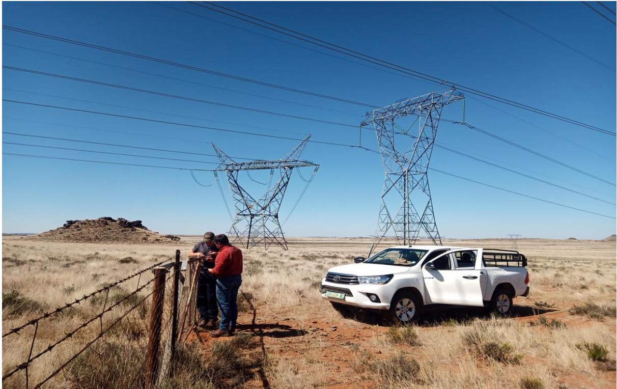
Figure 58: typical farm fence with existing pylons
