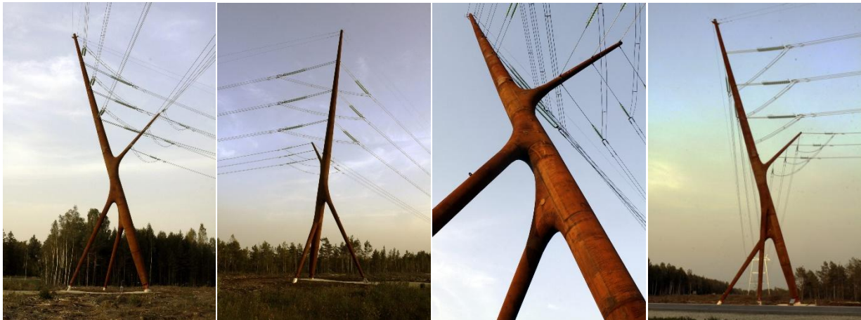
Figure 78: Soorebane ('bog-fox') high-voltage-pylon, Risti, Estonia Source: ahvenas, Altas Obscura
