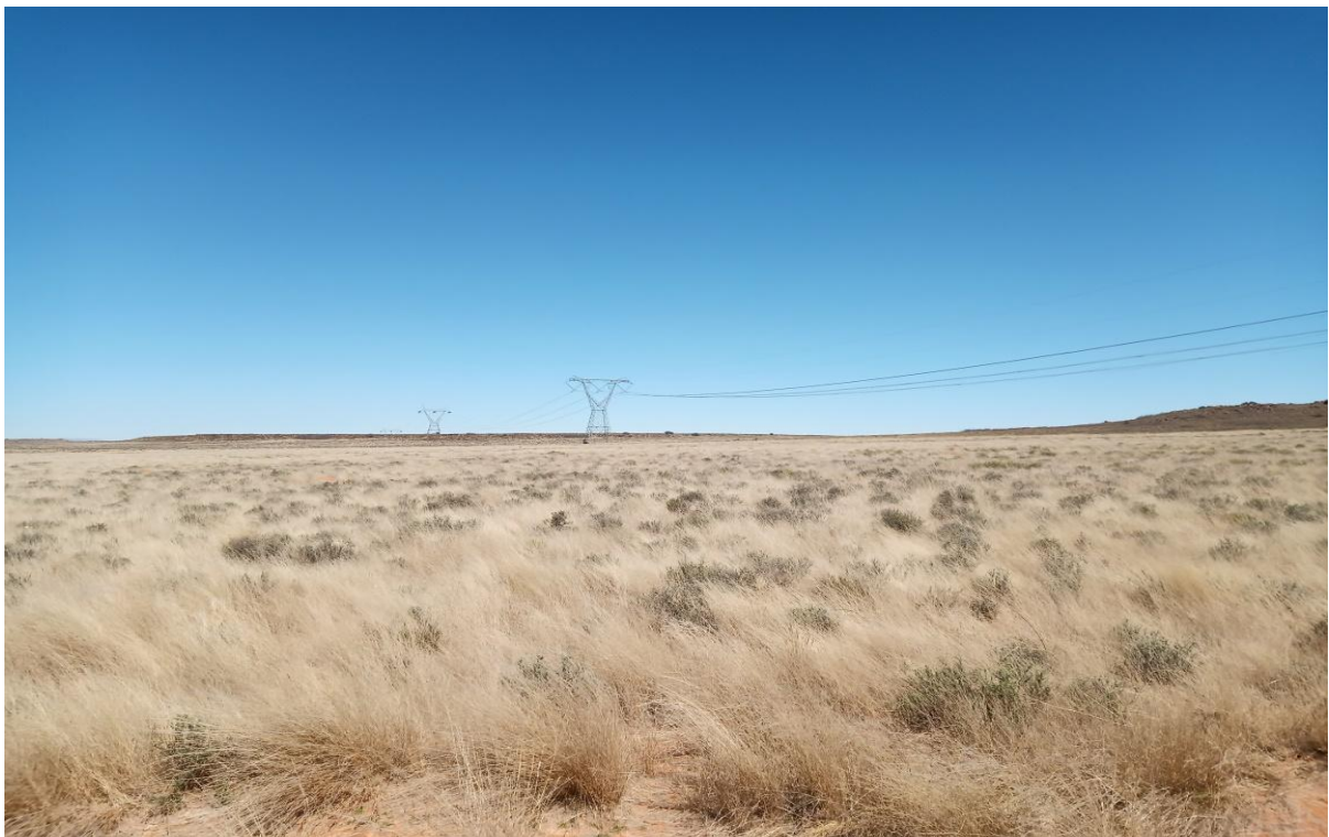
Figure 53: pylons lending a sense of scale
