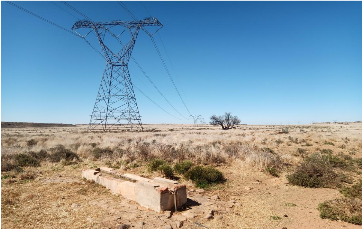
Figure 62: typical site view
