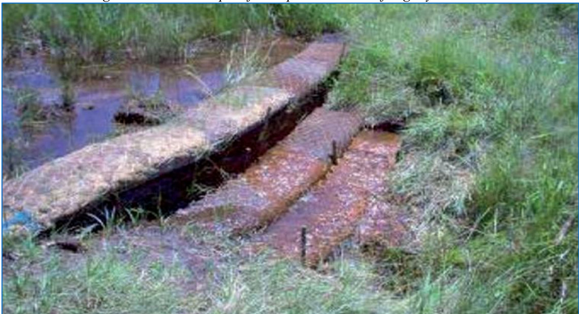
Figure A2.3: Example of fibre bags used to deactivate gully head erosion
