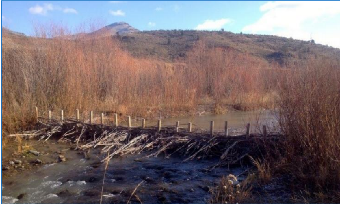
Figure A2.4: Example of soft engineering intervention – a stake and brush mattress structure
