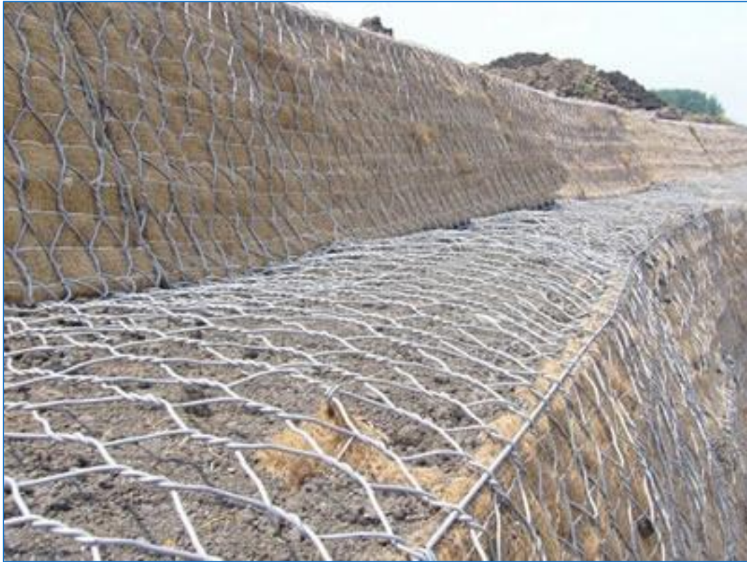
Figure A2.6: Example of stronger bank protection for bank stabilisation of higher velocity flow areas but allowing for vegetation establishment
