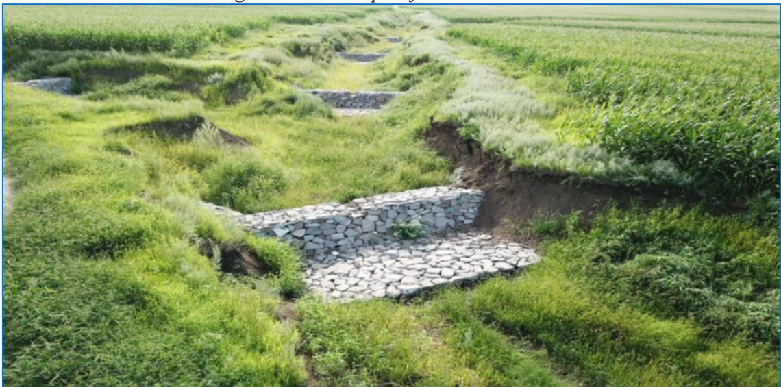
Figure A2.215: Example of multiple check dams for gully control
