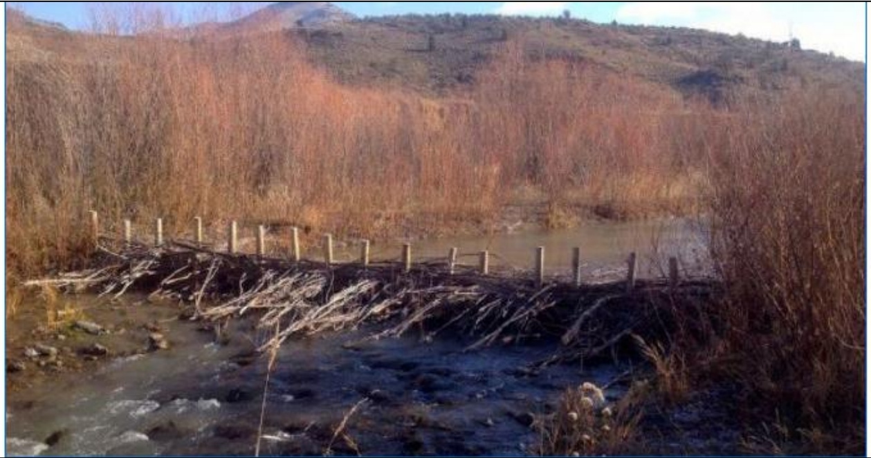
Figure 31: Example of soft engineering interventions- a stake brush mattress structure
