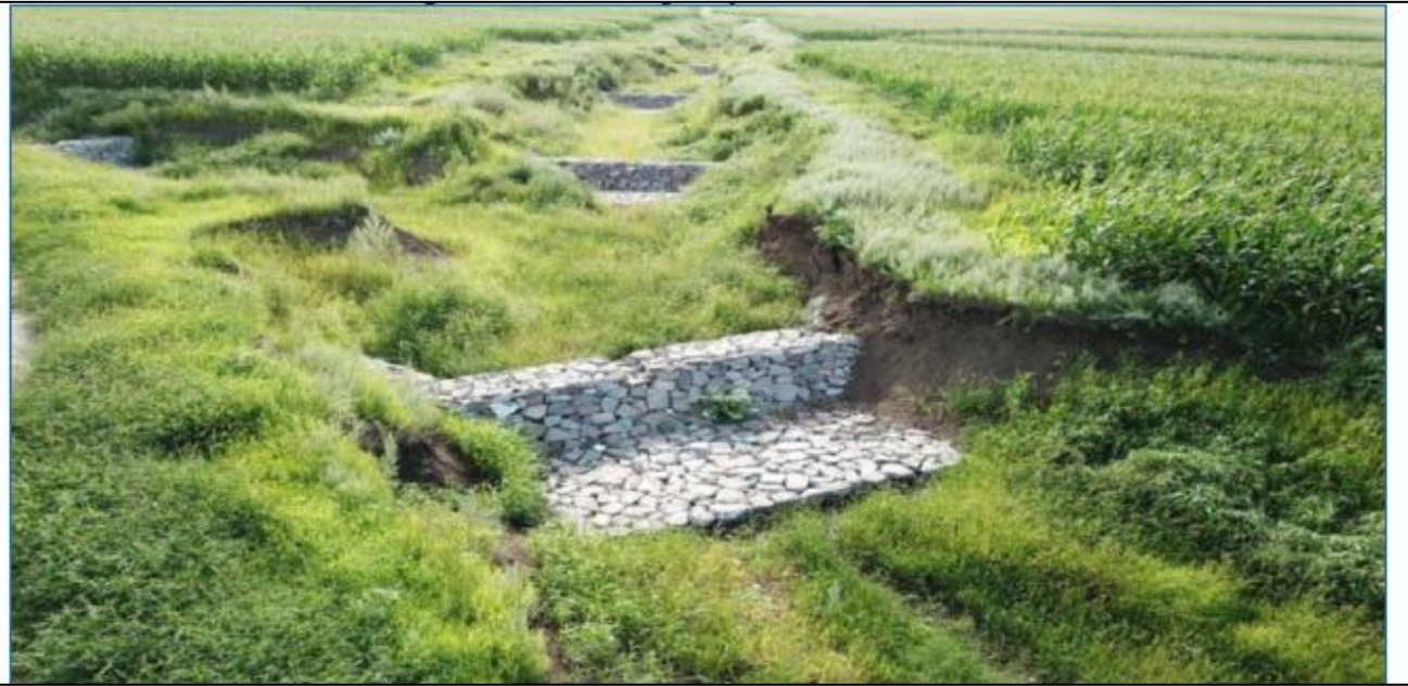
Figure 29: Example of multiple check dams for gully control.
