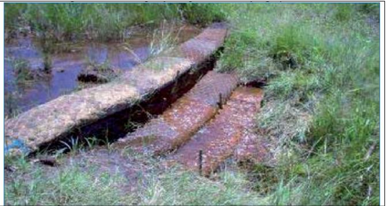
Figure 30: Example of fibre bags used to deactivate gully head erosion
