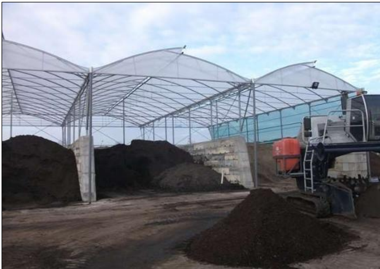
Figure 11: An Example of sludge storage bunds with concrete floors and translucent roof covers.
