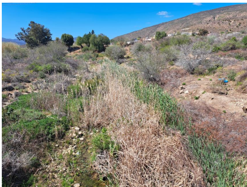
Figure 14: Photograph of the Nels River from Bridge 2664.
