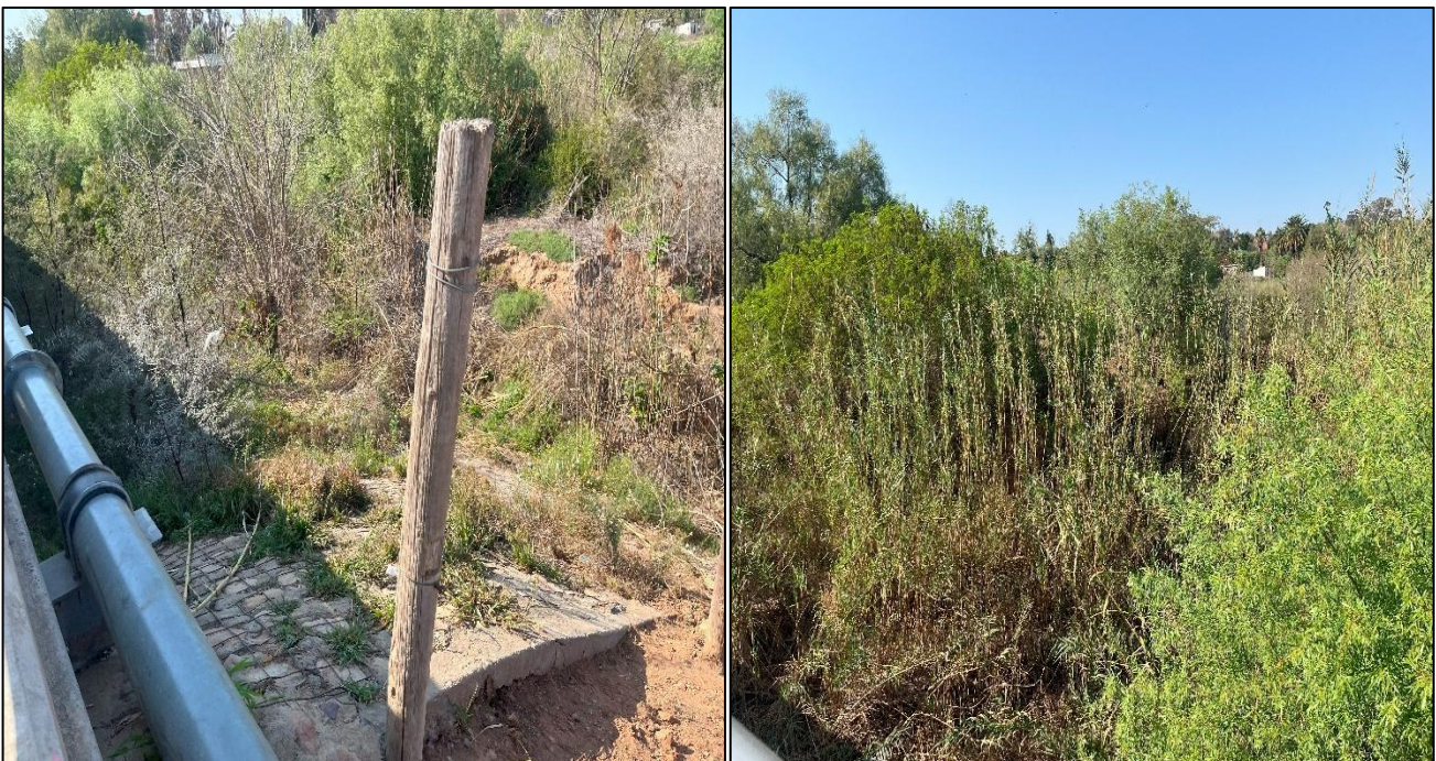
Figure 9 and 10: Nels River Bridge
