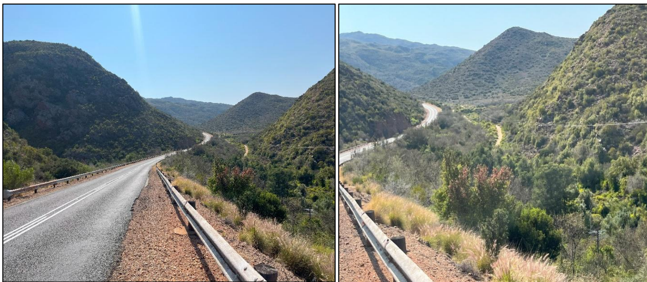
Figure 23 and 24: Vaarwel River Bridge.
