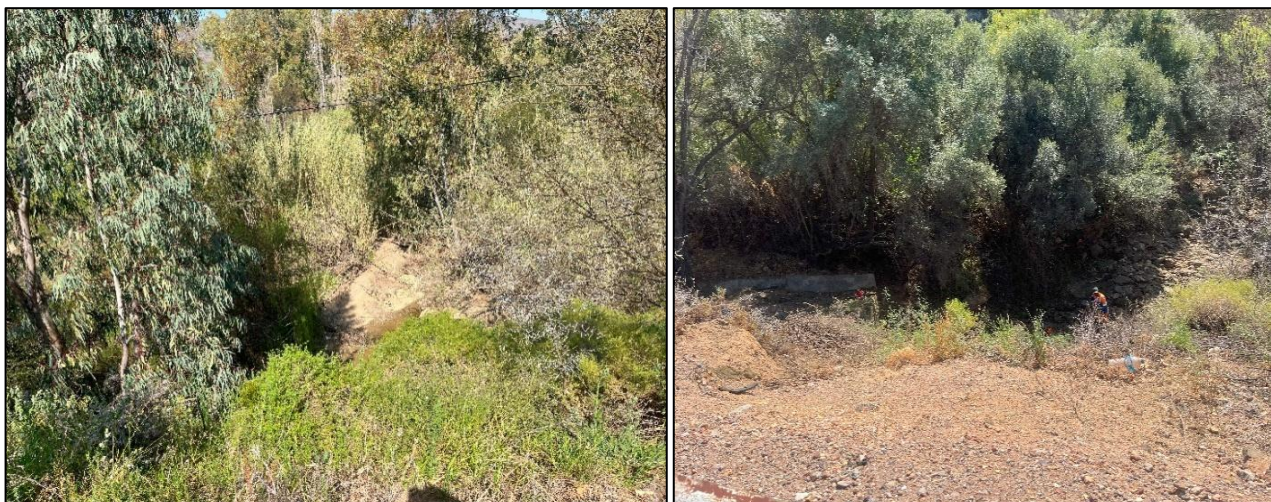
Figure 27 and 28: Wilge River Bridge.
