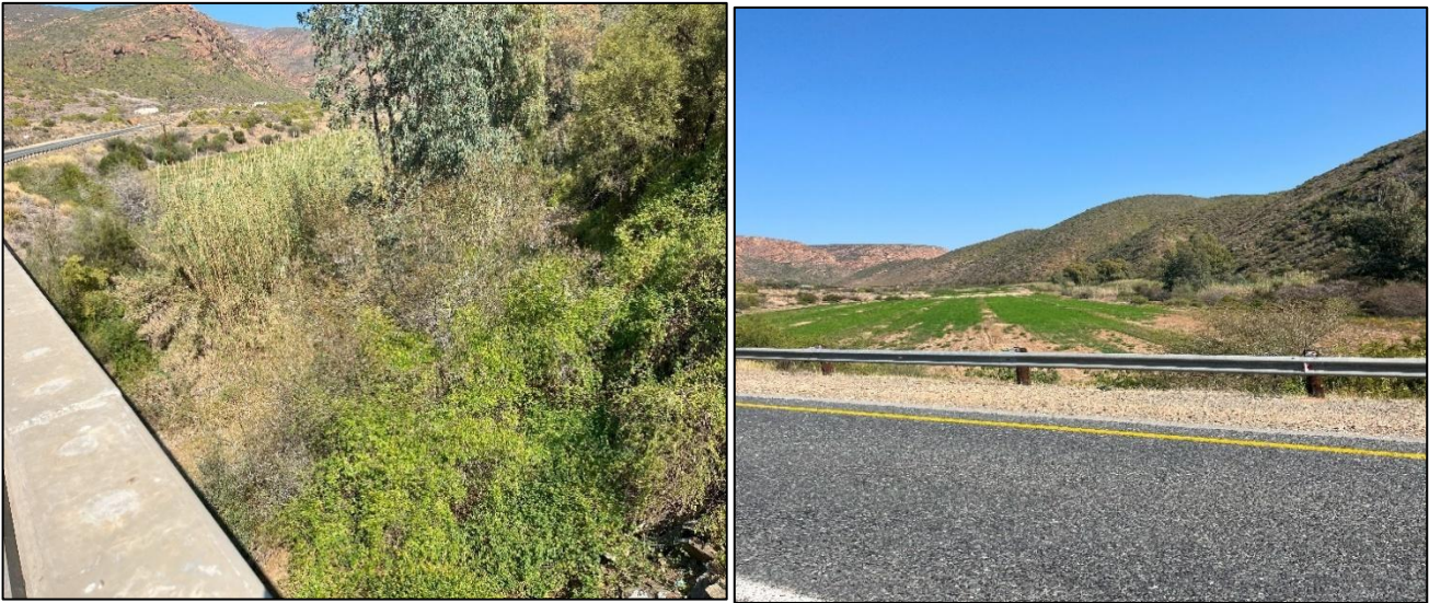
Figure 17 and 18: Huis River 1 Bridge.
