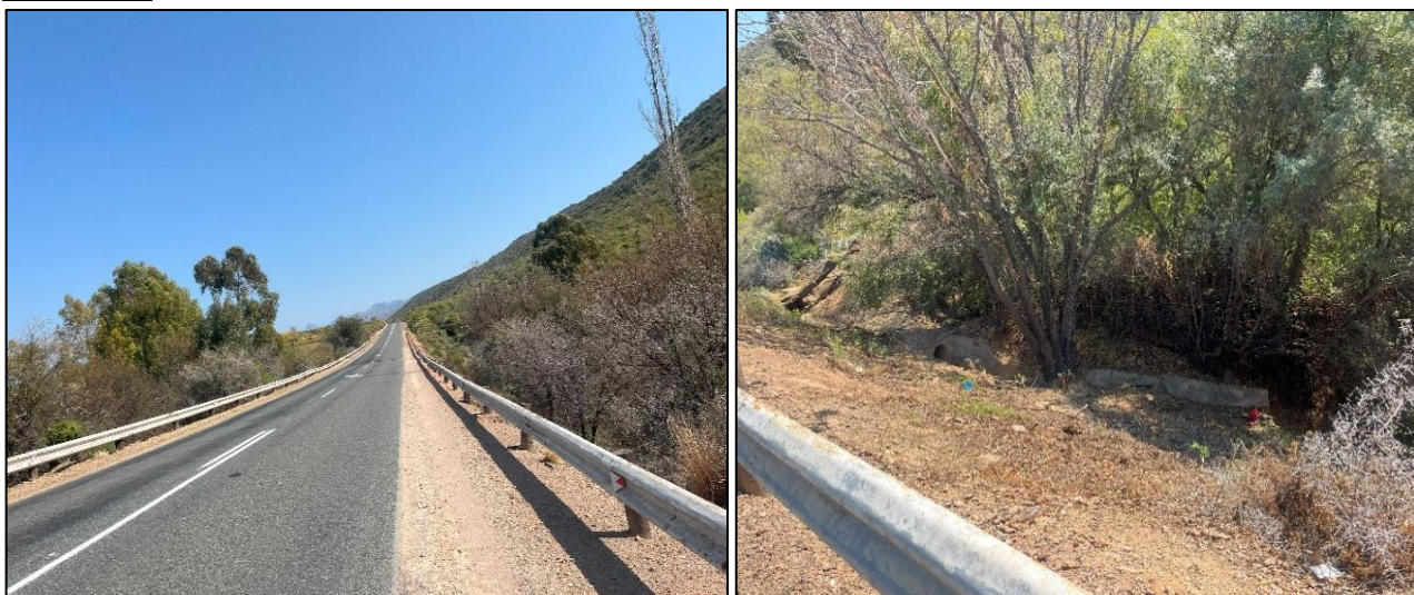
Figure 25 and 26: Wilge River Bridge.
