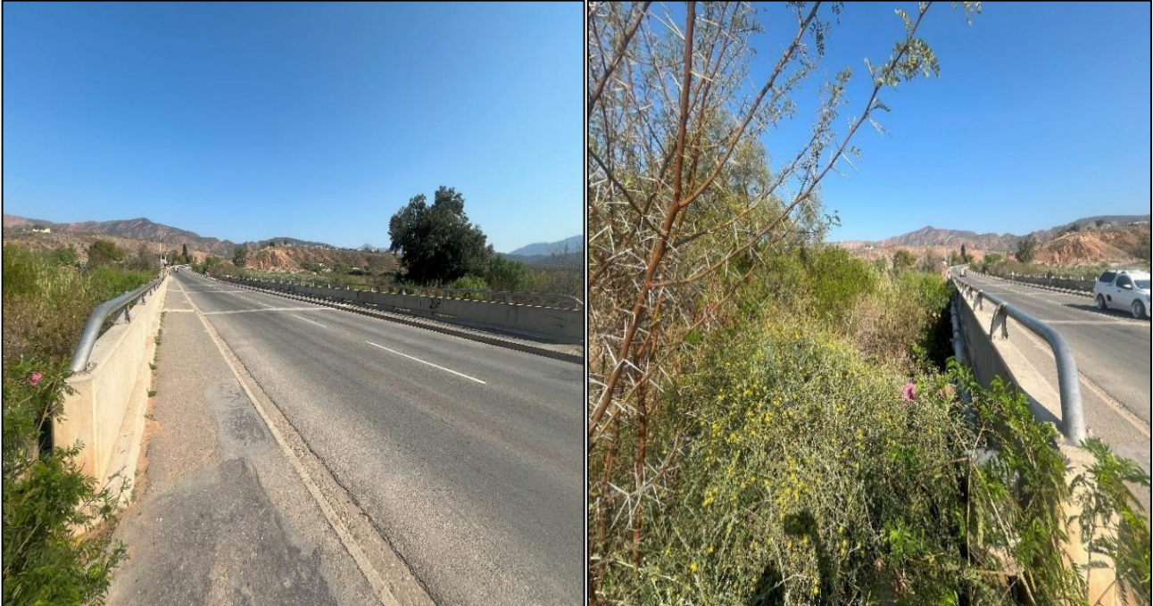
Figure 7 and 8: Nels River Bridge.
