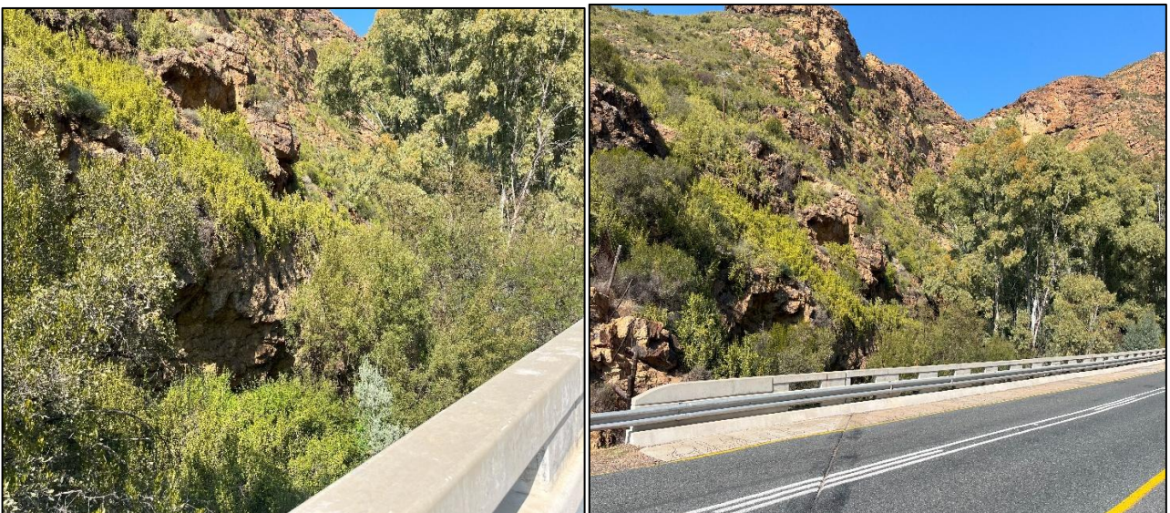
Figure 21 and 22: Huis River 2 Bridge.
