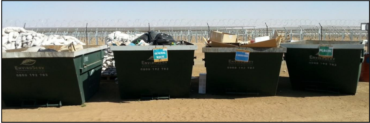
Image 42: Example of marked recycling skips within a site camp
