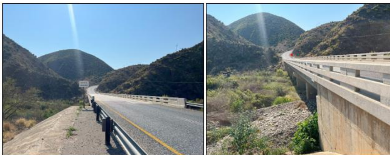
Figure 4: Gamka River Bridge.
