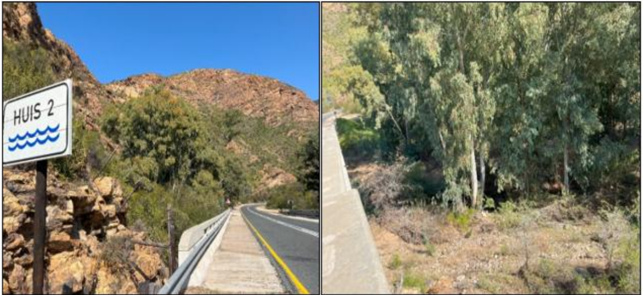
Figure 6: Huis River 2 Bridge.
