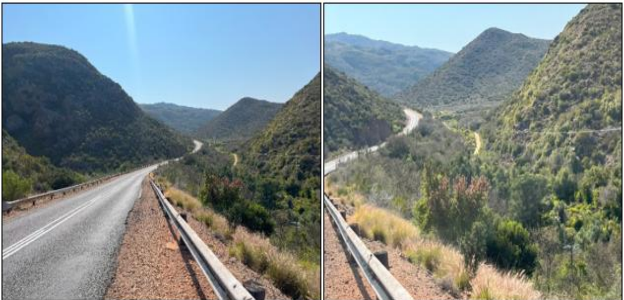
Figure 7: Vaarwel River Bridge.
