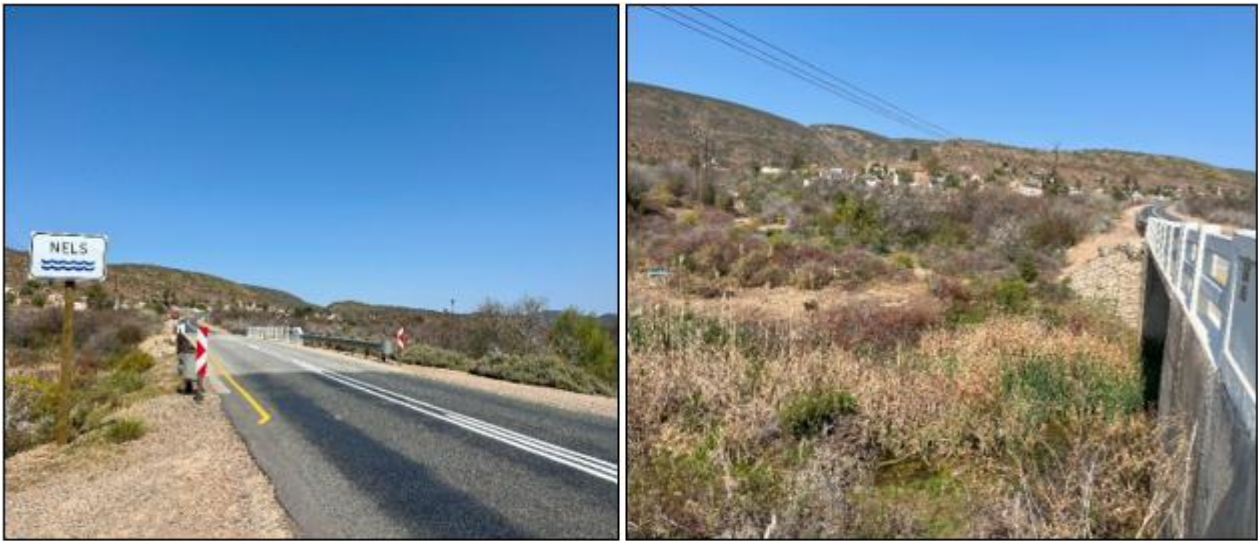
Figure 10: Nels River Bridge at Zoar.
