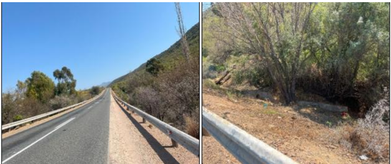
Figure 8: Wilge River Bridge.
