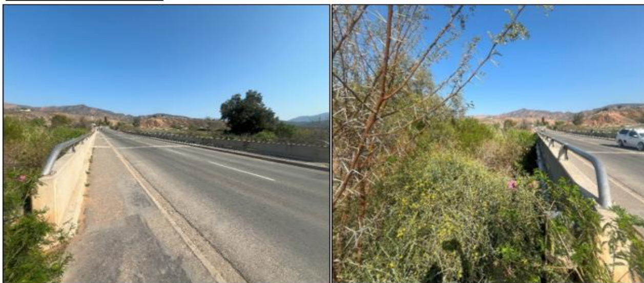
Figure 3: Nels River Bridge.
