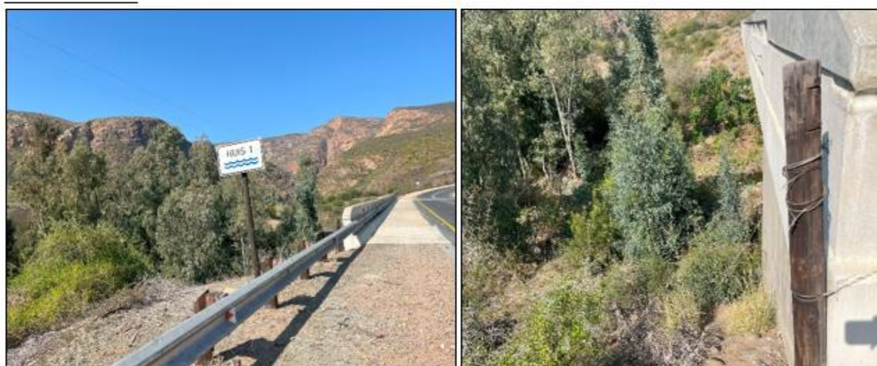
Figure 5: Huis River 1 Bridge.
