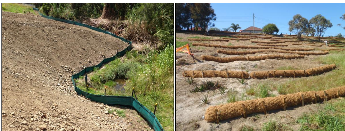
Figure 9: Examples of silt fences (left) and coir logs (right) used to trap sediment mobilised from steep slopes.
