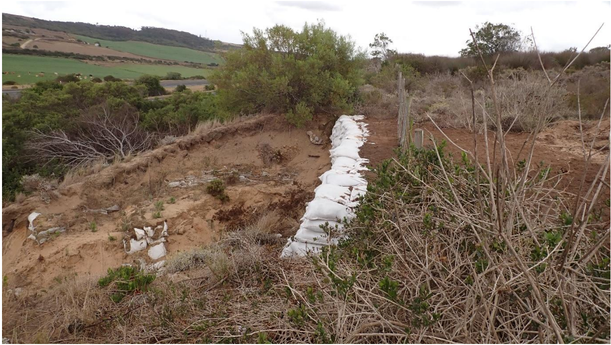
Figure 12B: Stormwater management structures across the central area of the property
