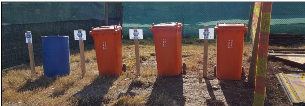
Image 1: Recycling system implemented on a construction site. Skips provided for general waste, plastic, cardboard and metal.
