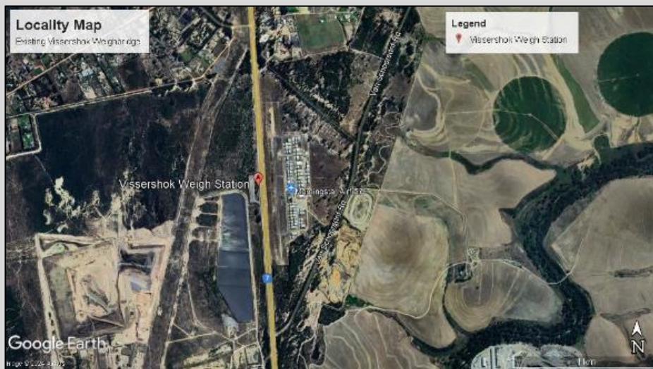
Figure 51. Existing Visserhok Weighbridge.
