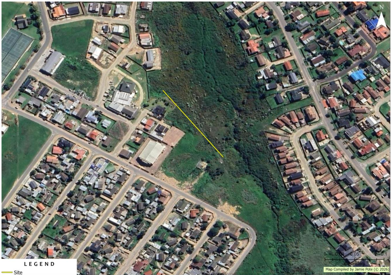
Figure 14: Aerial photo of the site (additional northern section).
