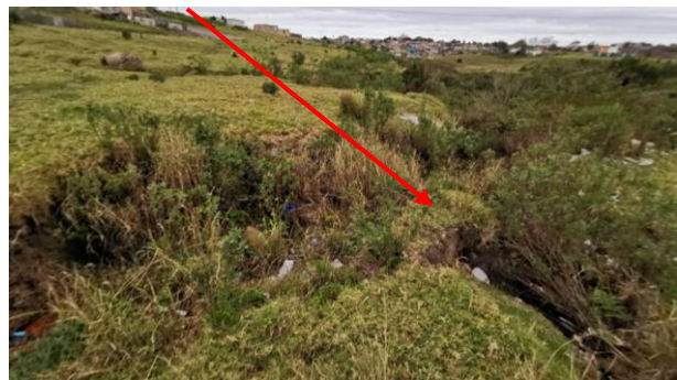
Figure 40: Eroded and polluted watercourse.
