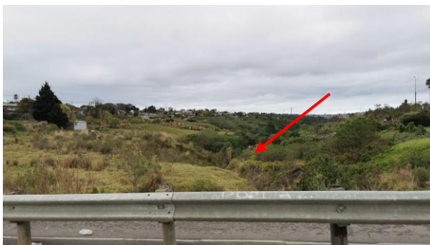
Figure 31: Watercourse bridge crossing.
