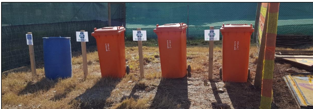
Image 2: Recycling system implemented on a construction site. Lidded bins provided for general waste, plastic, cardboard, and metal.
