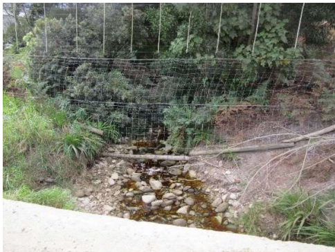
Upstream – looking away from culvert
