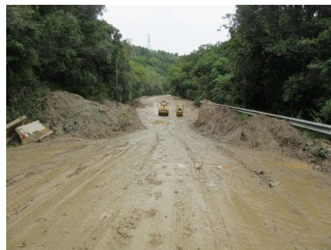
Road MR00355 at km 3.77; upstream on LHS. Backfilling in progress.
