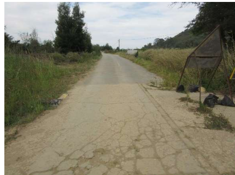
Road DR1791 at km 1.59; upstream on RHS.
