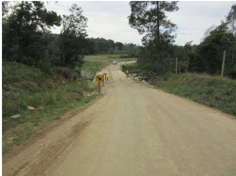
Road DR01633 at km 3.35; upstream on LHS.
