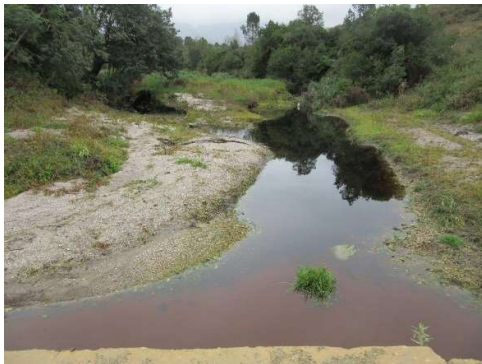
Upstream – looking away from culvert
