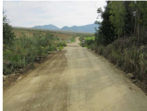
Road DR1639 at km 1.63; upstream on RHS.
