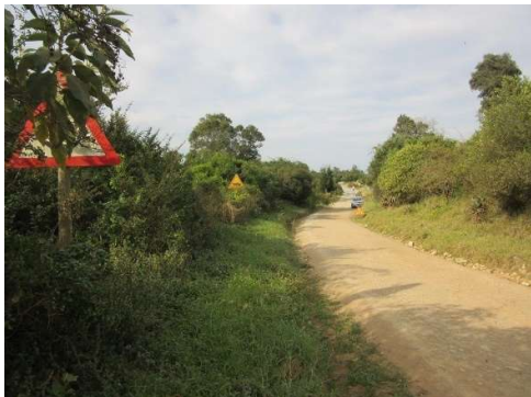
Road DR1791 at km 1.59; upstream on RHS.
