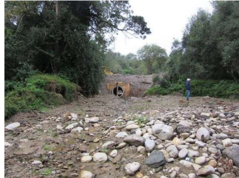
Downstream – looking towards culvert
