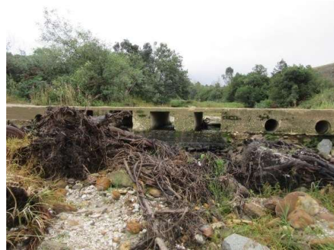
Downstream – looking towards culvert
