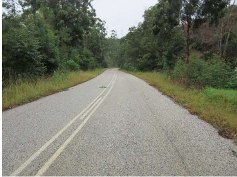
Road MR00355 at km 3.00
