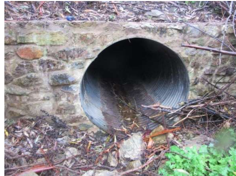
Head fall and culvert inlet
