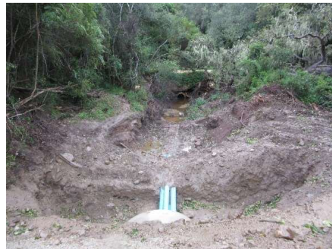
Upstream – looking away from culvert
