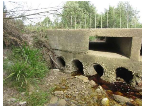
Upstream – looking towards culvert
