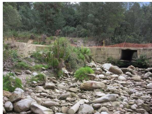
Downstream – looking towards culvert
