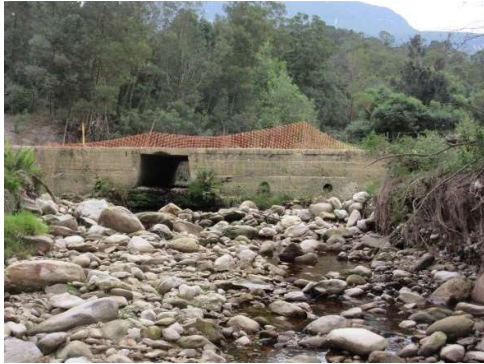
Downstream – looking towards culvert
