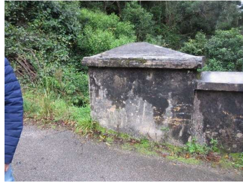
Image of existing end-block on opposite side of the bridge
