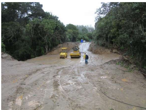
Road MR00355 at km 3.77; upstream on RHS. Backfilling in progress.
