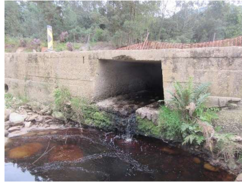
Downstream – looking towards culvert
