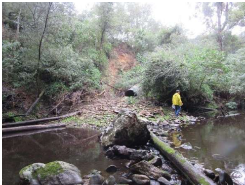
Downstream – looking towards culvert
