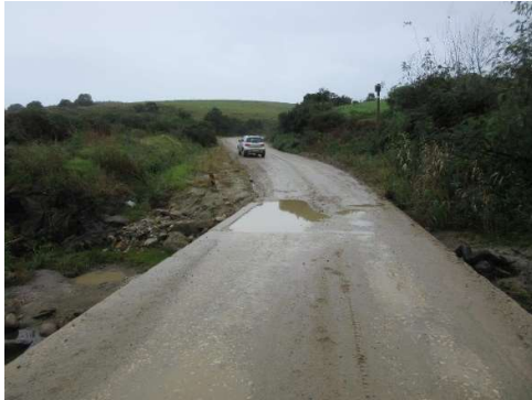
Road DR1602 at km 8.48; upstream on RHS.
