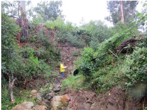
Upstream – looking towards culvert
