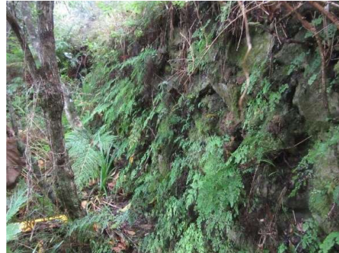
Close-up view of rock wall
