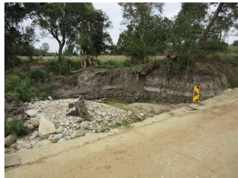
Downstream – looking away from culvert
