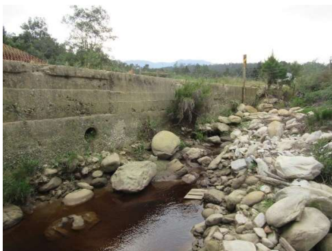
Downstream – looking towards culvert
