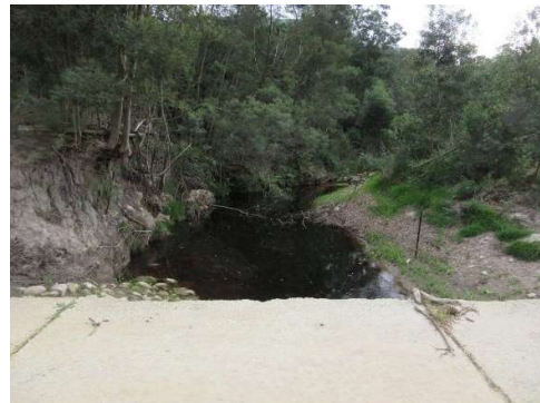
Upstream – looking away from culvert
