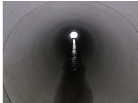
Inside newly installed pipe culvert
