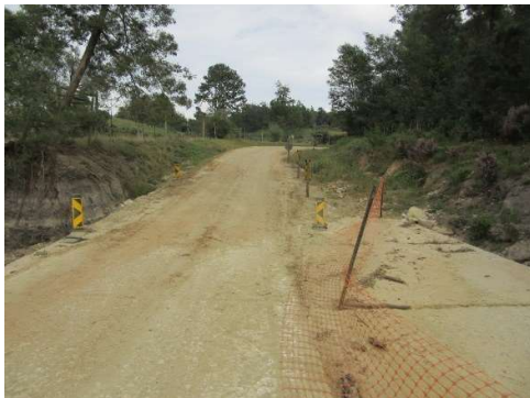
Road DR01633 at km 3.35; upstream on RHS.
