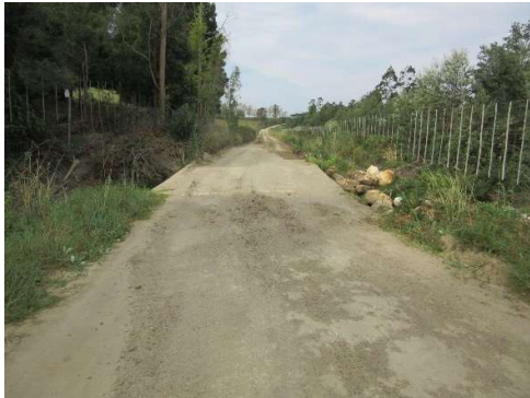
Road DR1639 at km 1.63; upstream on LHS.
