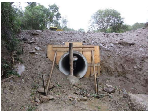
Downstream – looking towards culvert. Headwall construction in progress.
