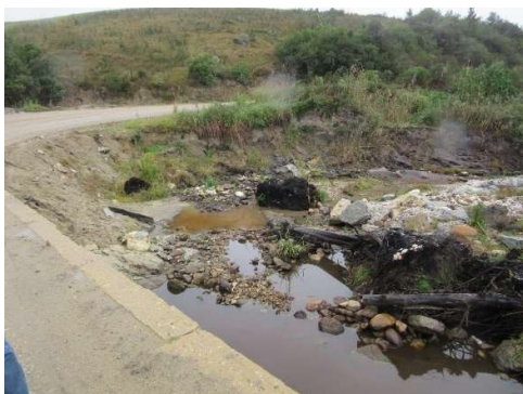
Downstream – looking away from culvert
