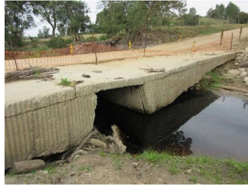
Upstream – looking towards culvert
