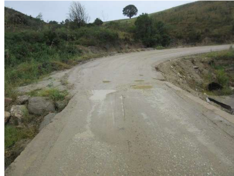
Road DR1602 at km 8.48; upstream on LHS.
