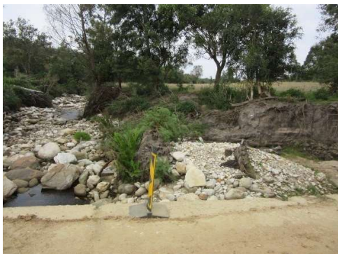
Downstream – looking away from culvert
