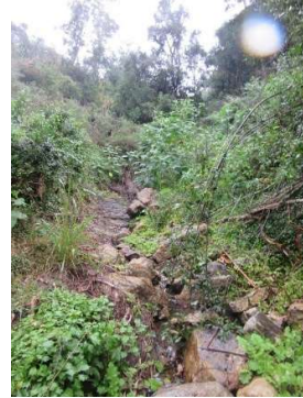
Upstream – looking away from culvert
