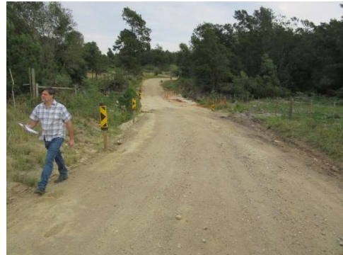
Road DR01633 at km 3.35; upstream on RHS.
