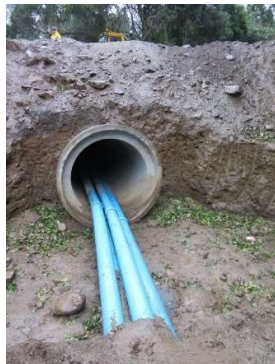
Upstream – looking towards culvert
