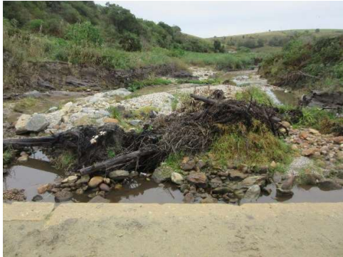
Downstream – looking away from culvert
