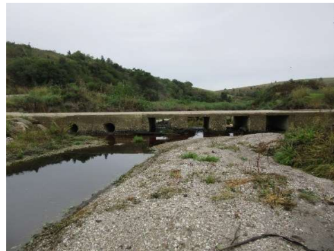
Upstream – looking towards culvert
