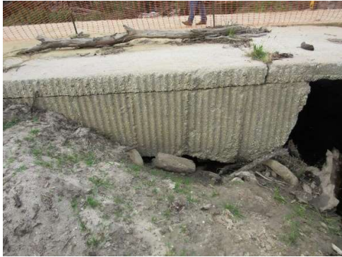
Upstream – looking towards culvert
