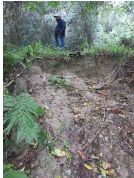
2.2m high rock wall on the edge of the road
