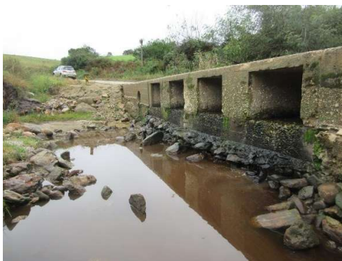
Downstream – looking towards culvert
