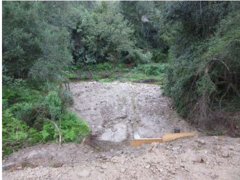
Downstream – looking away from culvert
