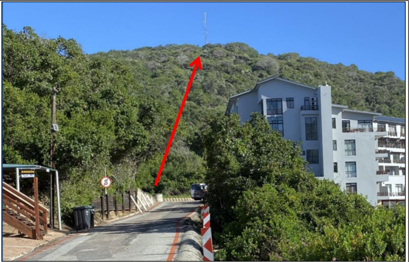
Figure 19: Approximate route of proposed pipeline (red arrow) through coastal thicket towards the WWTW. (Extract from M. Berry's Botanical Assessment)
