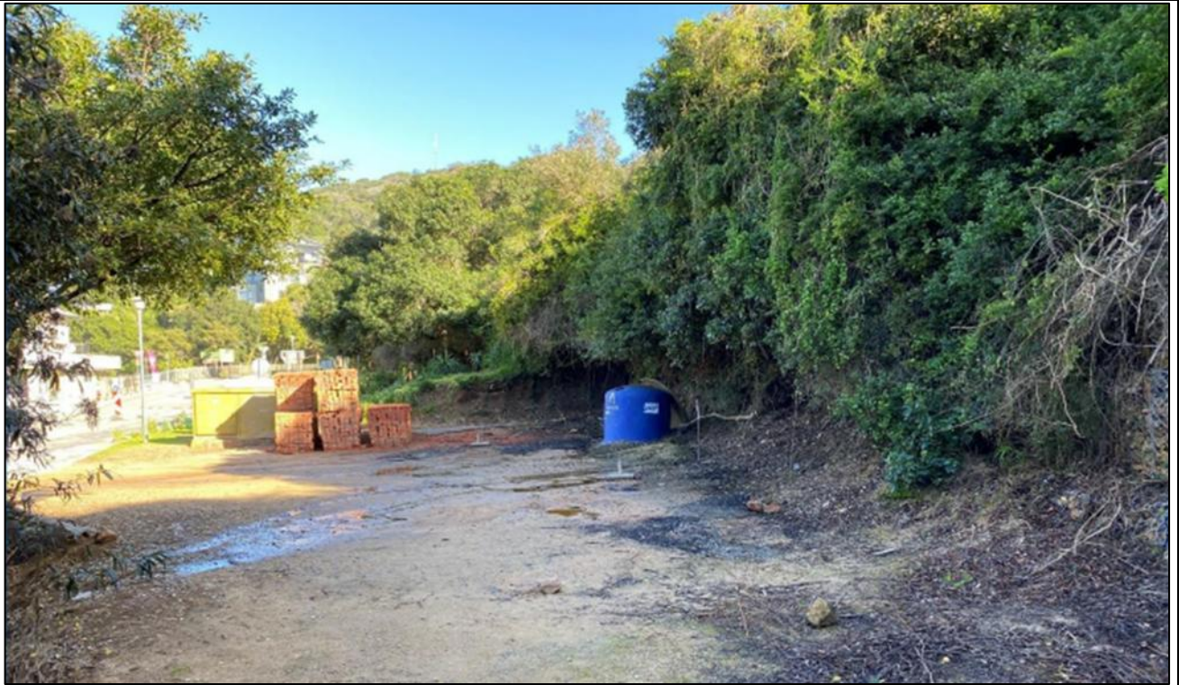
Figure 21: Site proposed for the new pump station PS4. (Extract from M. Berry's Botanical Assessment)
