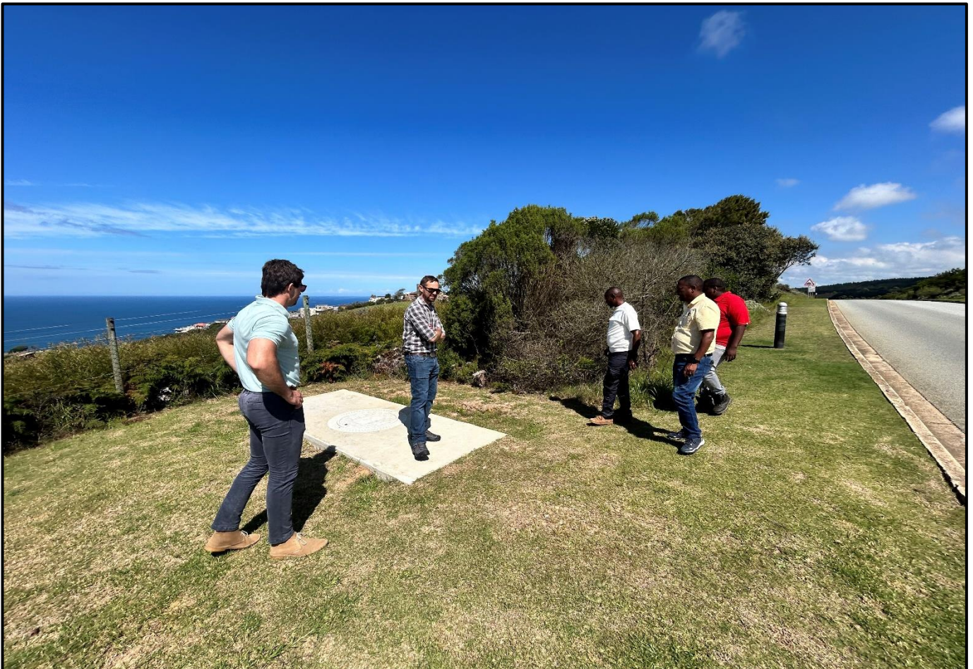
Image 14: Connection point of pipeline.
