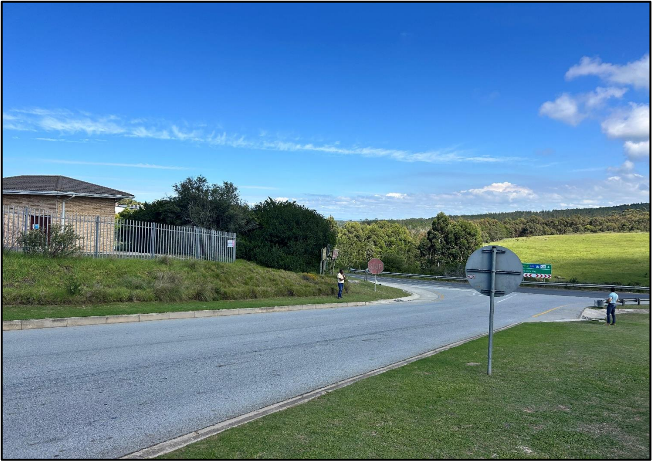
Image 7: Connection point of pipeline at Estate Boulevard / Oubaai Road.
