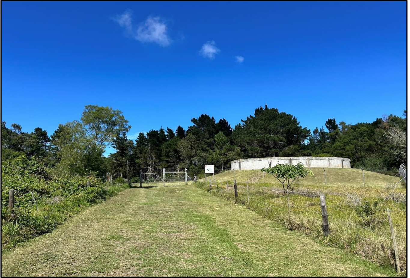
Image 3: Entrance road and Oubai Reservoir site.
