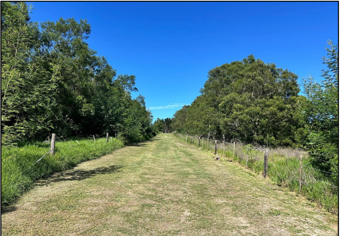
Image 2: Entrance road to Oubaai Reservoir site.
