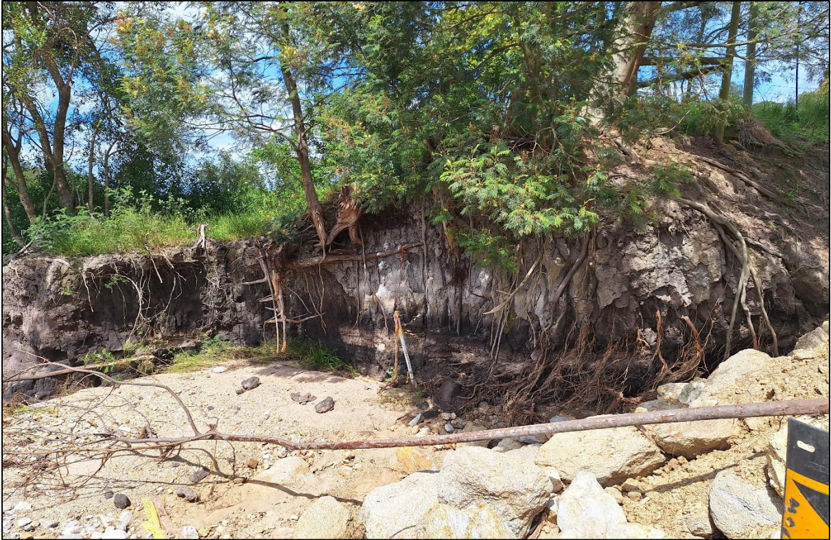
Plate 8: Photograph of the bank erosion on the downstream side of the causeway resulting from altered channel morphology and the effect of Wattle Tree roots on river banks
