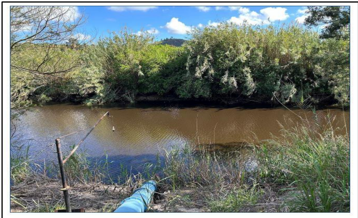
Figure 12: Moordkuil River with one of the water abstraction pipes.
