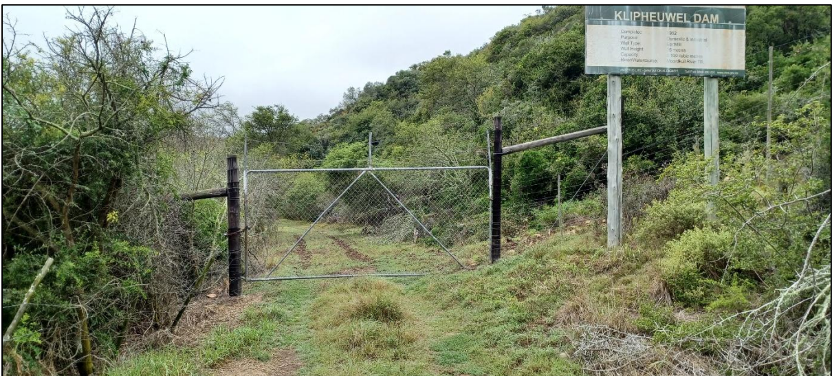
Plate 8: Access Road built on banks of HGM 3 to the base of the Klipheuwel Dam wall.
