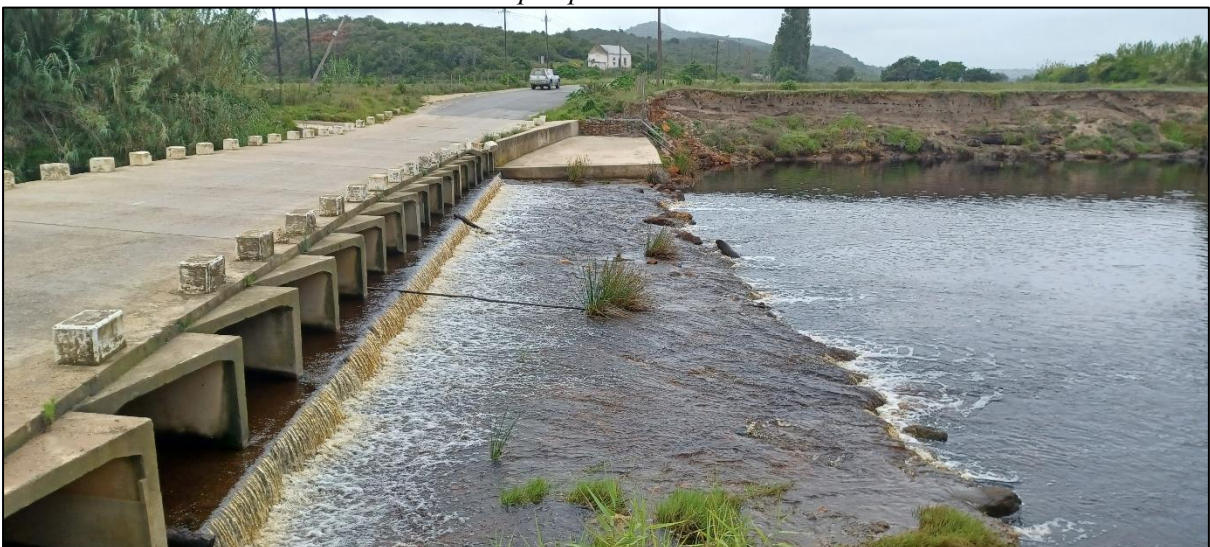
Plate 4: A photograph taken of the current road crossing the Moordkuil River, which prevents salt water ingress from the estuary downstream. Note the steep eroded east bank.
