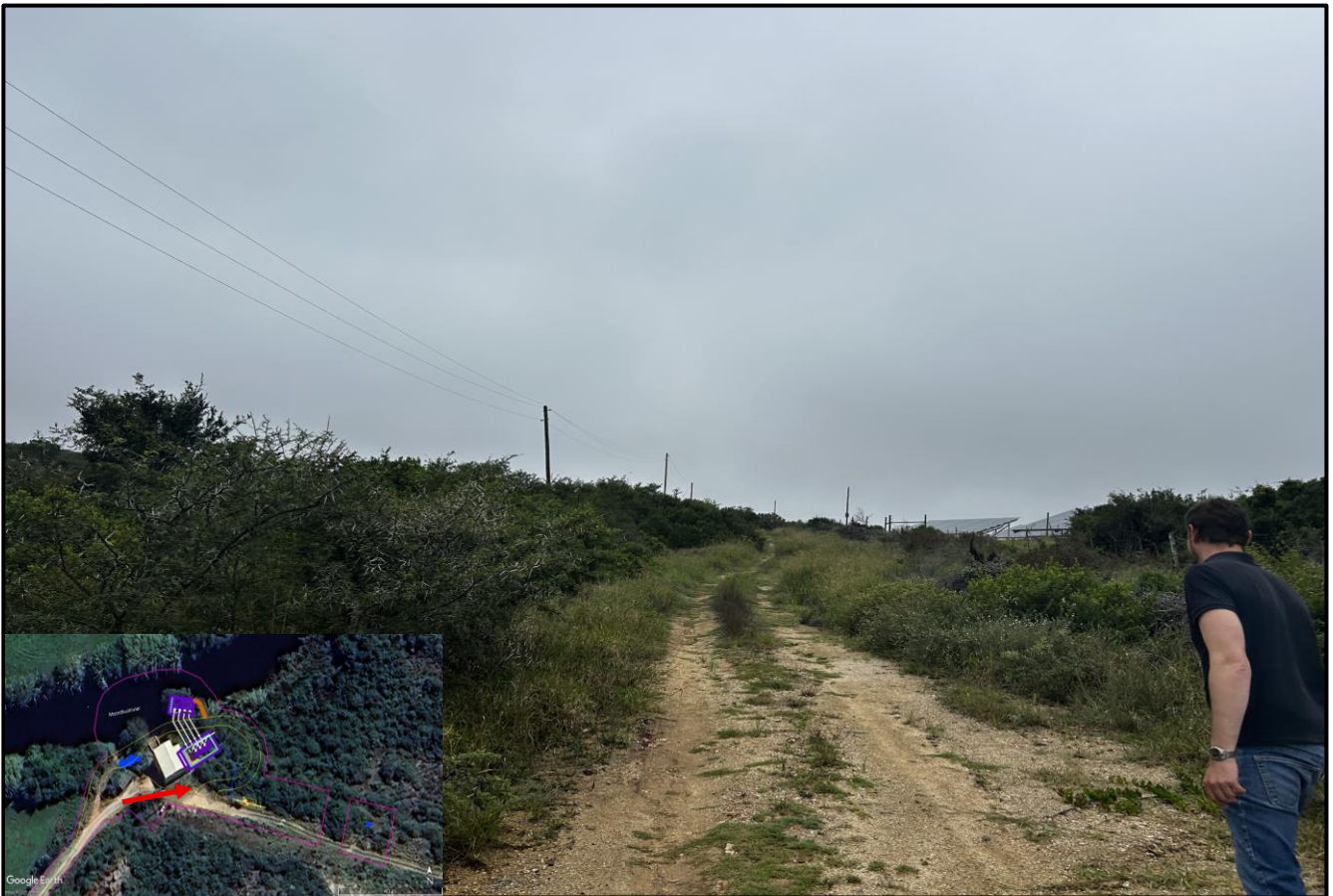
Figure 13: Access road, area where water meter chamber will be installed, and area where cement access road to the pump station will be installed (28 February 2025).
