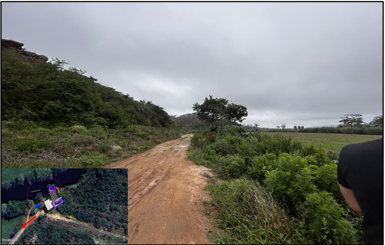
Figure 19: Road where a new cement access road will be installed (28 February 2025).
