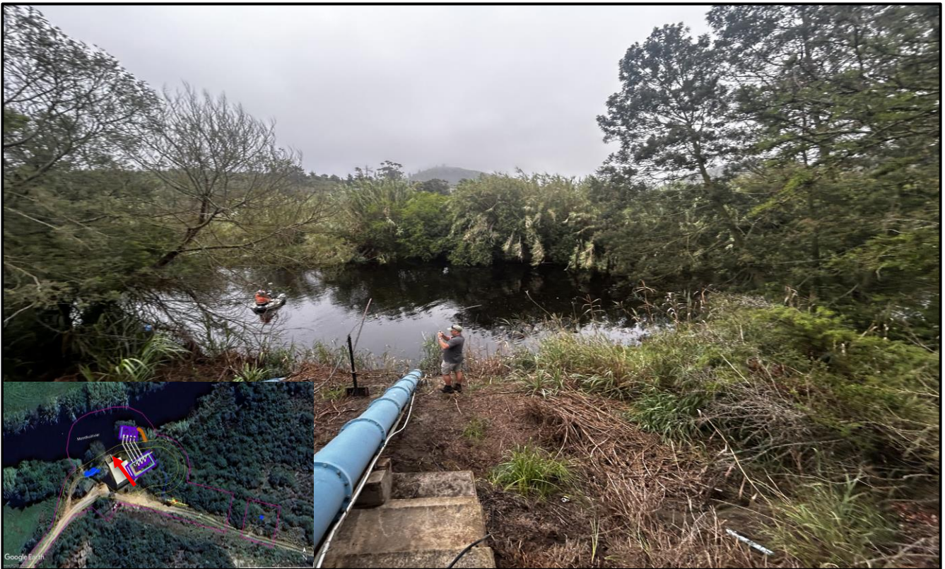
Figure 11: View of the Moordkuil River from the Moordkuil Pump Station (28 February 2025).
