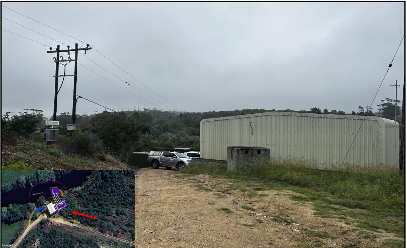
Figure 14: Access road, area where water meter chamber will be installed, and area where cement access road to the pump station will be installed (28 February 2025).
