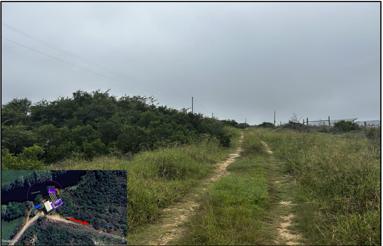
Figure 15: Access road and area where valve chamber will be installed (28 February 2025).
