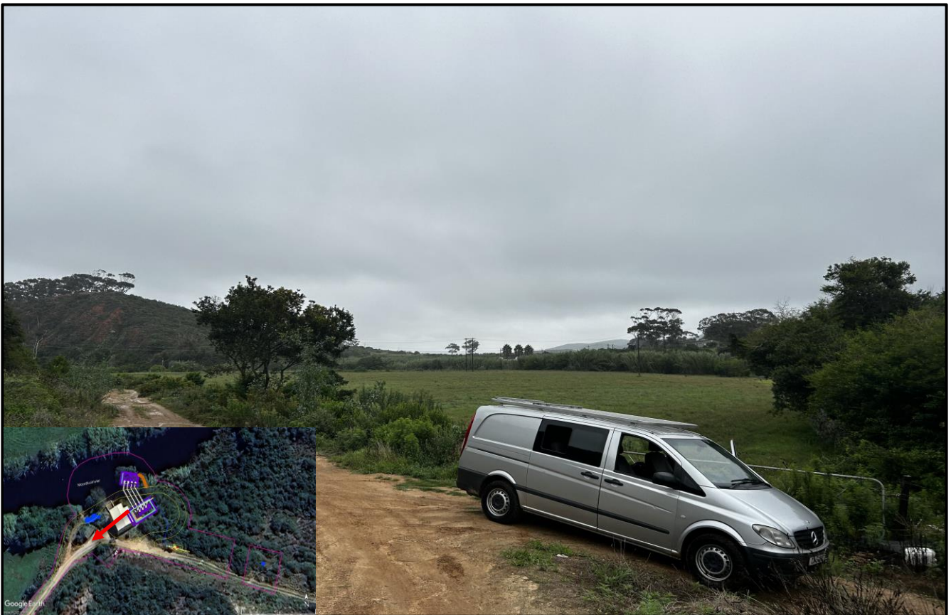
Figure 18: Road where a new cement access road will be installed (28 February 2025).
