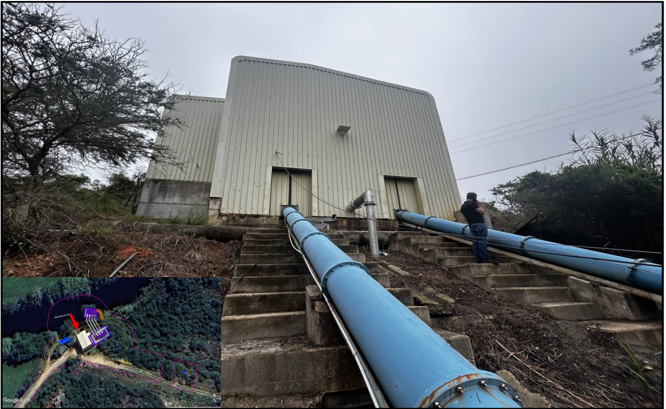
Figure 10: Southern view of the existing Moordkuil Pump Station (28 February 2025).
