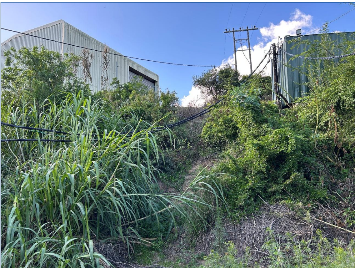
Figure 5-2: Embankment on western side of pump station, covered by pioneer shrubs and reeds.
