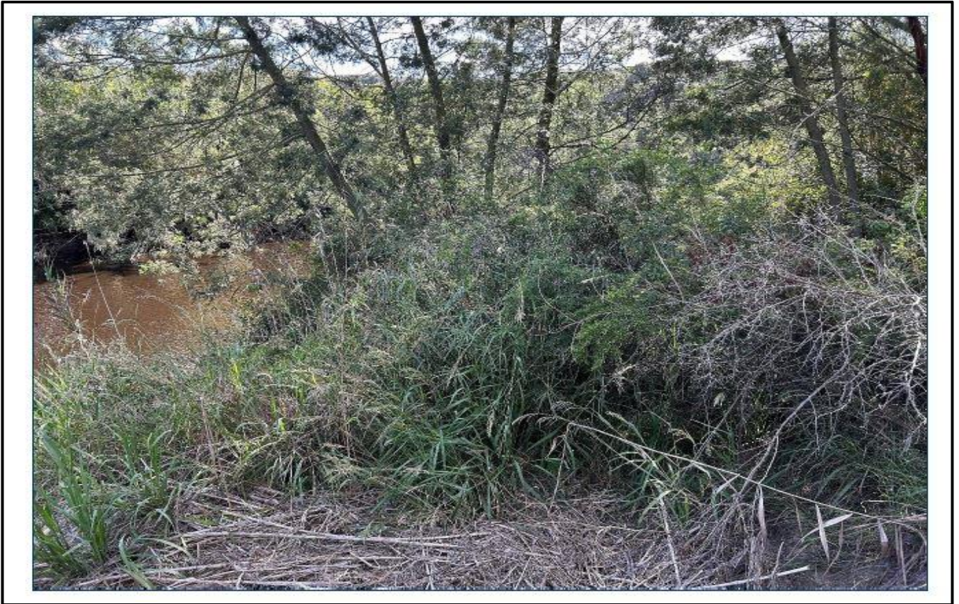
Figure 9: Degraded vegetation on eastern side of pump station.
