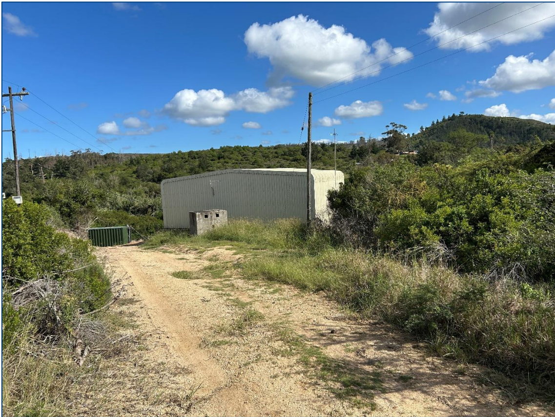
Figure 5-3: Thicket on eastern side of pump station and position of temporary access to construction site.
