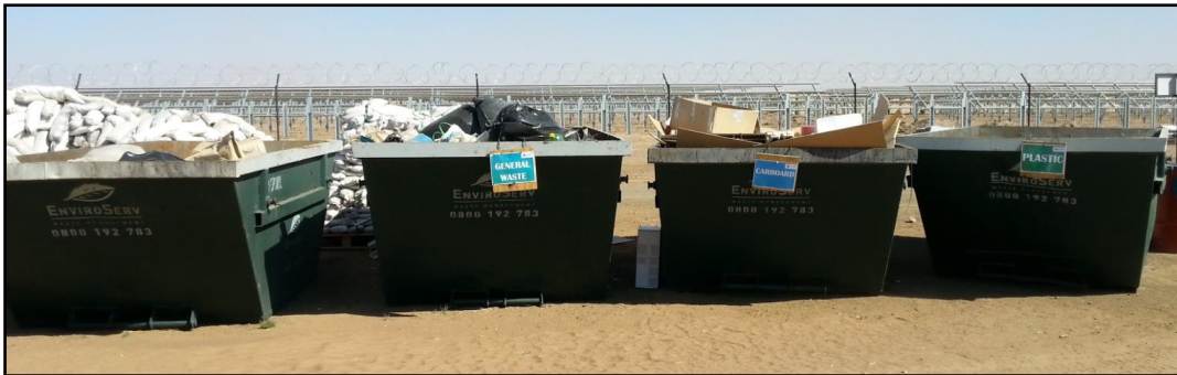
Image 1: Recycling system implemented on a construction site. Skips provided for general waste, plastic, cardboard and metal.
