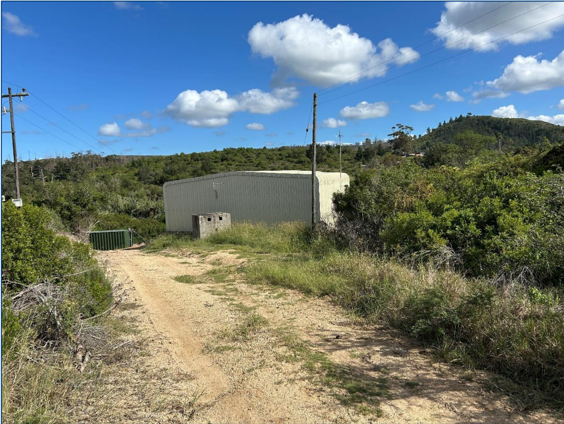
Figure 5-3: Thicket on eastern side of pump station and position of temporary access to construction site.
