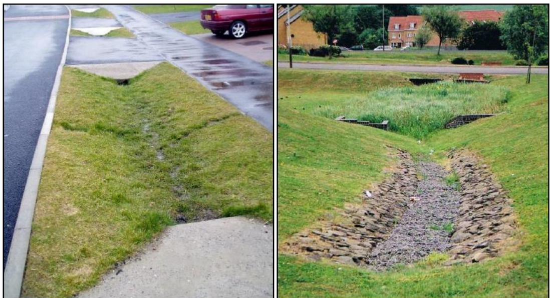
Figure 20. Examples of soft infrastructure incorporated into the stormwater management design.
