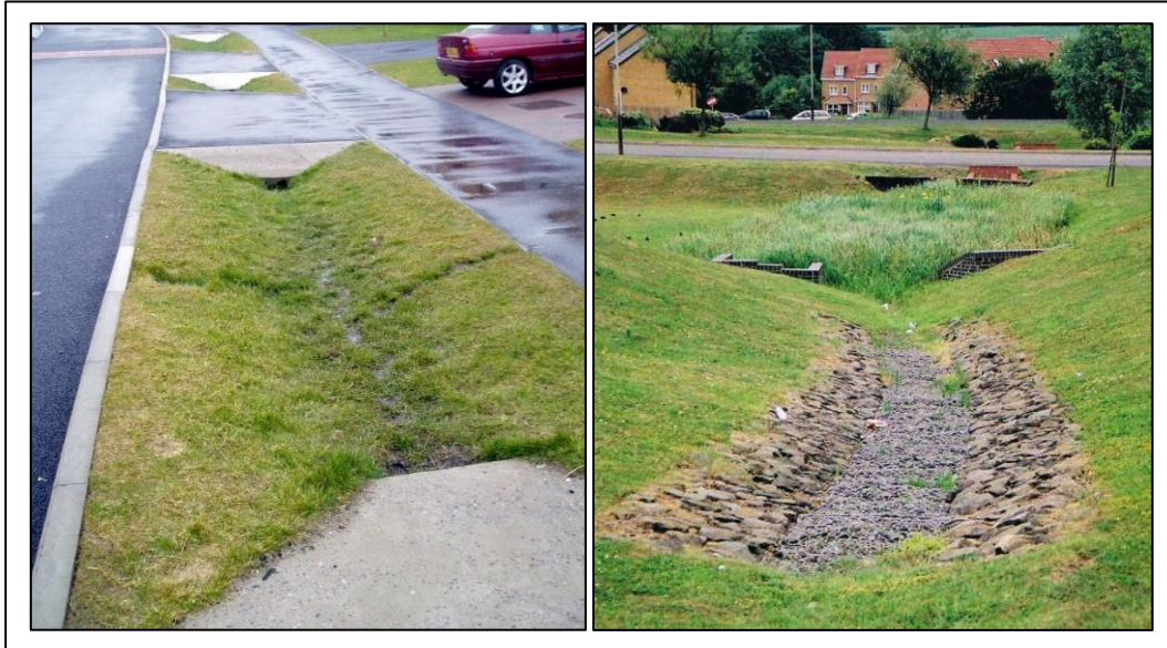
Figure 27: Examples of soft infrastructure incorporated into the stormwater management design
