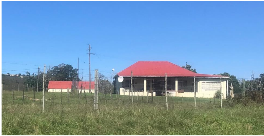
Building A – probably mid 20 th C farm house Suggested grading: IIIC - contextual value
