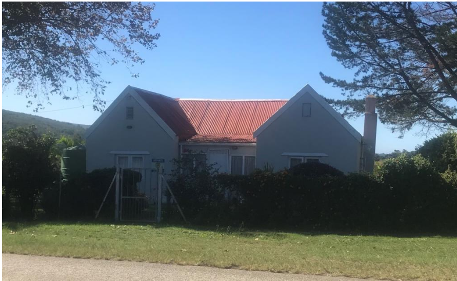
Building D – Two bay cottage, probably mid to late 19 th C, alterations to windows and steep visible Suggested grading: IIIC – contextual value
