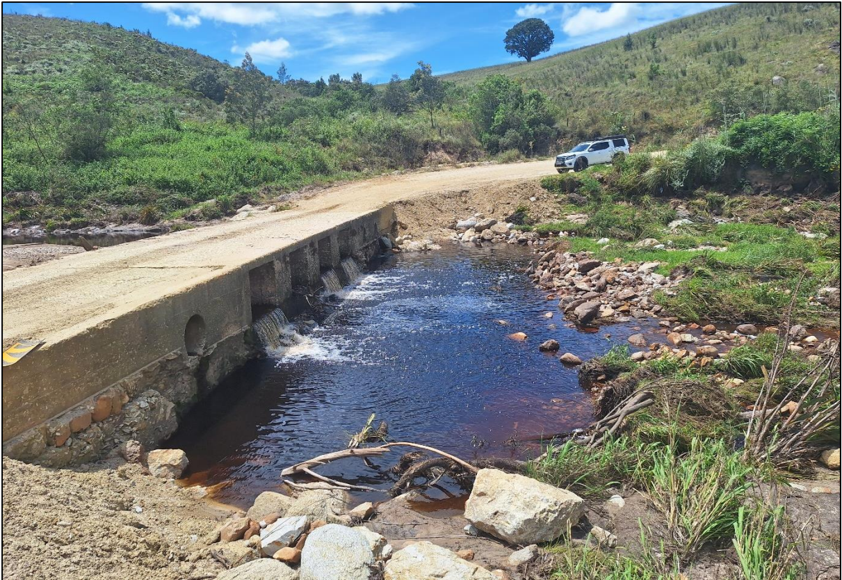
Plate 10: Photograph showing the culvert confining flows resulting in scouring of the river bed downstream and erosion of the banks
