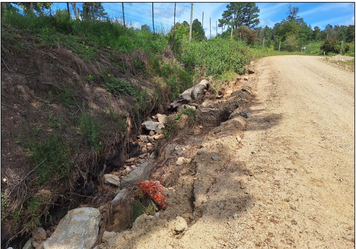
Plate 9: Photograph of road side stormwater drain causing sedimentation of the river
