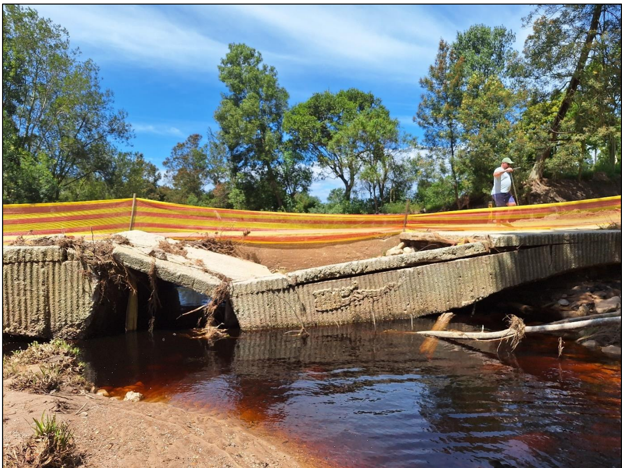
Plate 1: Photograph of the collapsed Site 4 causeway on the DR1633 Jonkersberg Road (km 3.35) over the Varings River in Jonkershoek
