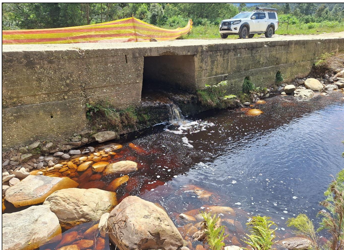
Plate 7: Photograph of the single small culvert at the site 4 causeway resulting in confined flow and scour downstream
