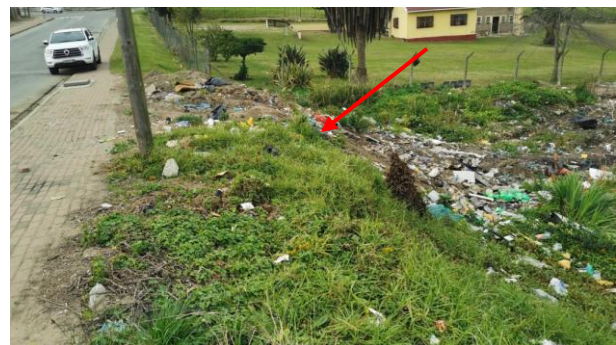
Figure 32: Discharge point at watercourse crossing.
