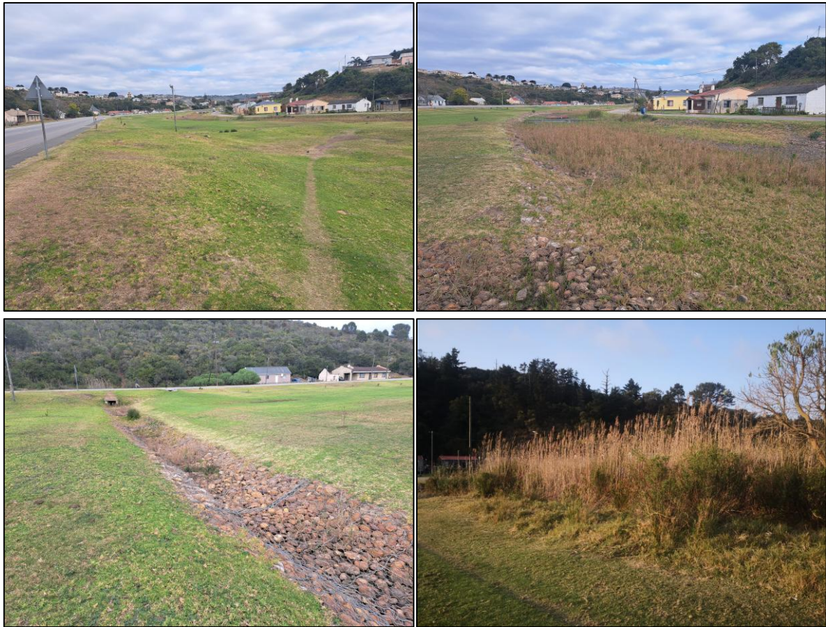
Figure 9: Photographs of the grassed area adjacent to the canal (top left), the canal lined with open concrete pavers (top right), a stormwater channel leading from Amy Searle Street down towards the canal (bottom left) and a patch of remnant wetland vegetation in close proximity to Amy Searle Street (bottom right).
