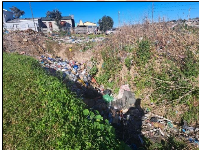
Figure 4: An example of an existing stormwater outlet with no headwall and no erosion protection.
