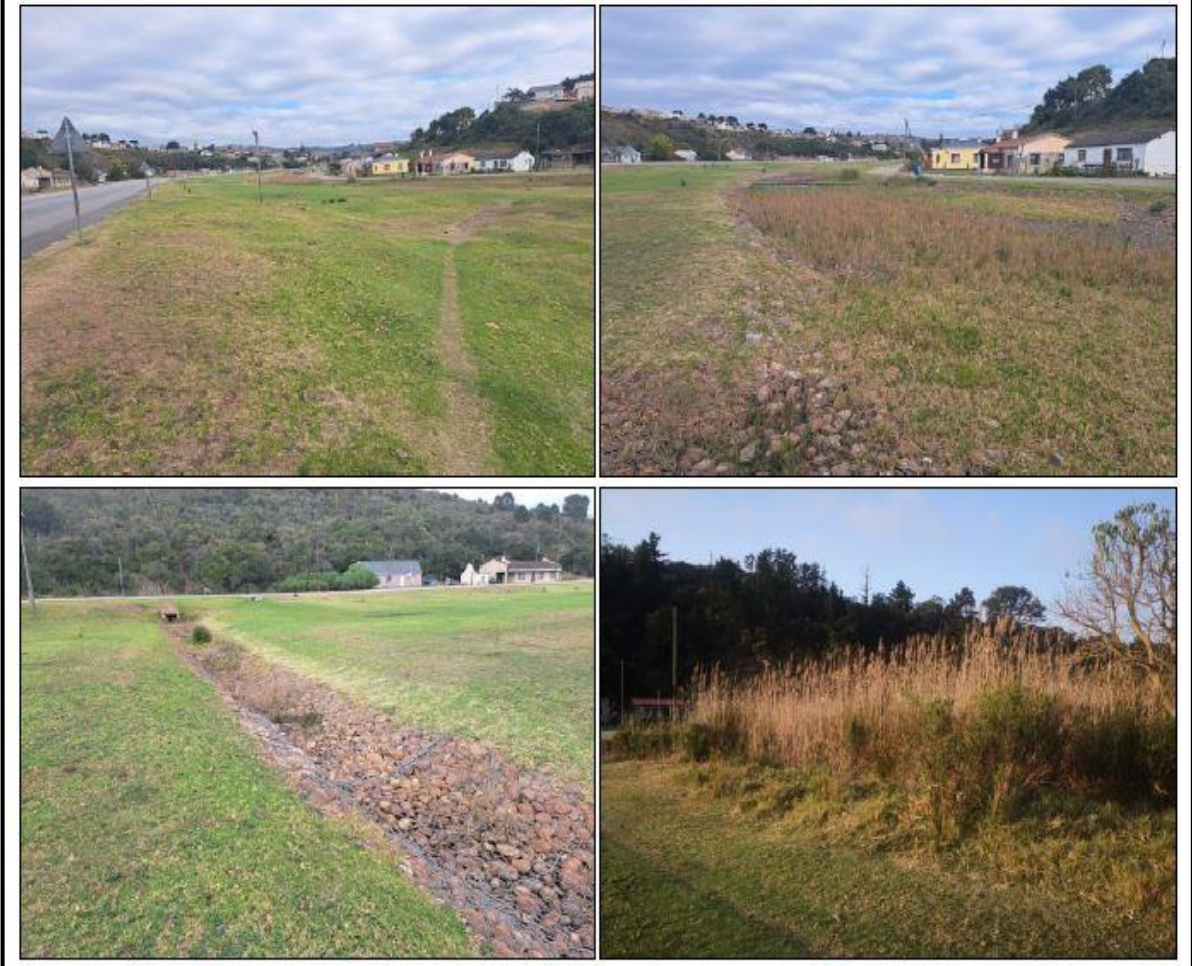
Figure 15: Photographs of the grassed area adjacent to the canal (top left), the canal lined with open concrete pavers (top right), a stormwater channel leading from Amy Searle Street down towards the canal (bottom left) and a patch of remnant wetland vegetation in close proximity to Amy Searle Street (bottom right).
