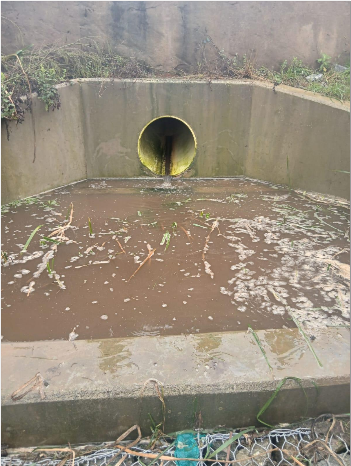
Figure 4: OWWTW Stormwater outlet structure free of blockages
