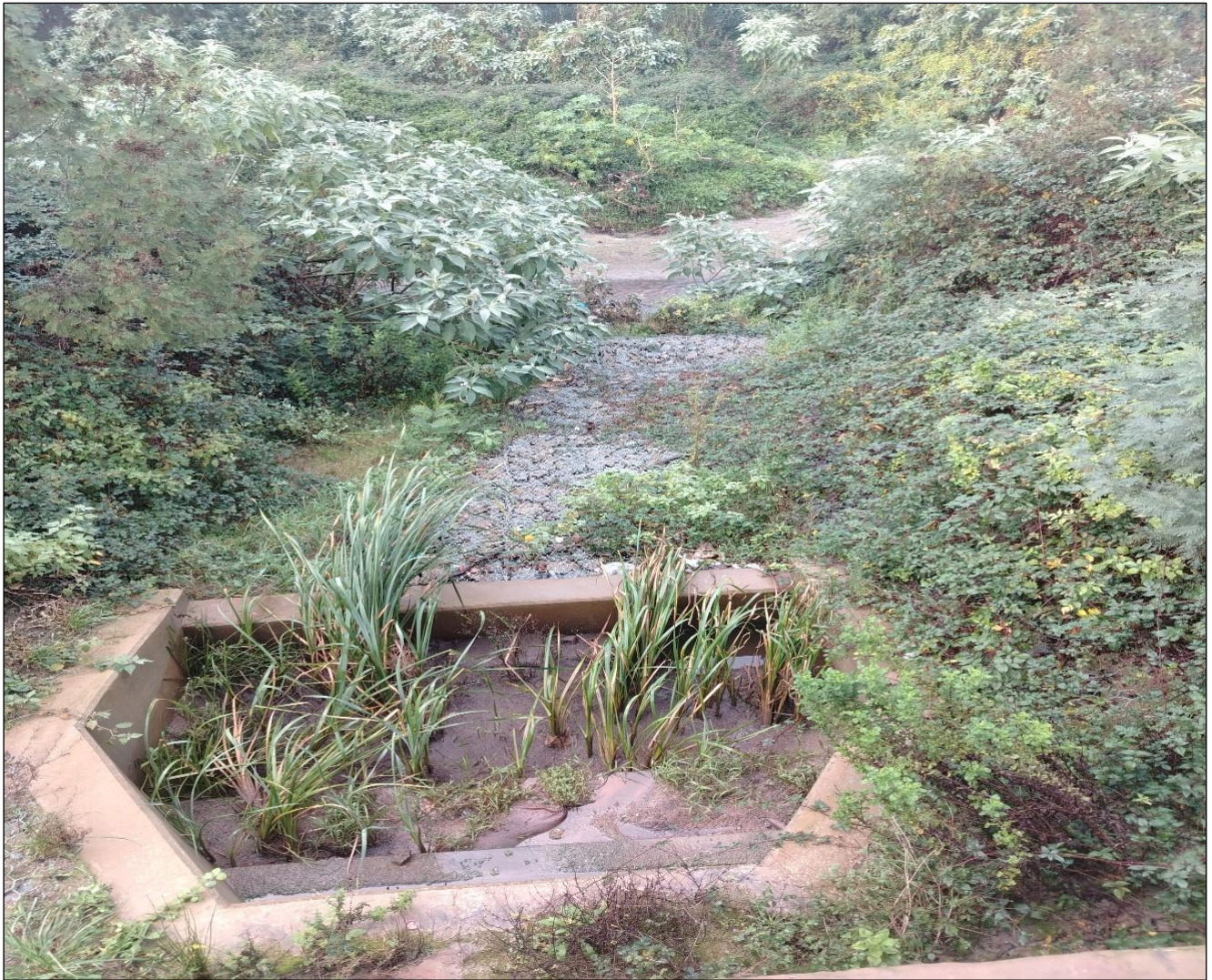
Figure 1: OWWTW Retention Pond – Prior to Alien Clearing
