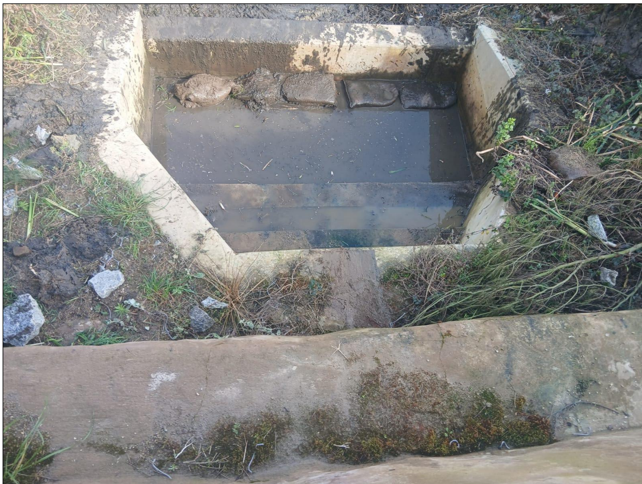
Figure 3: OWWTW Detention Pond – After Alien Clearing
