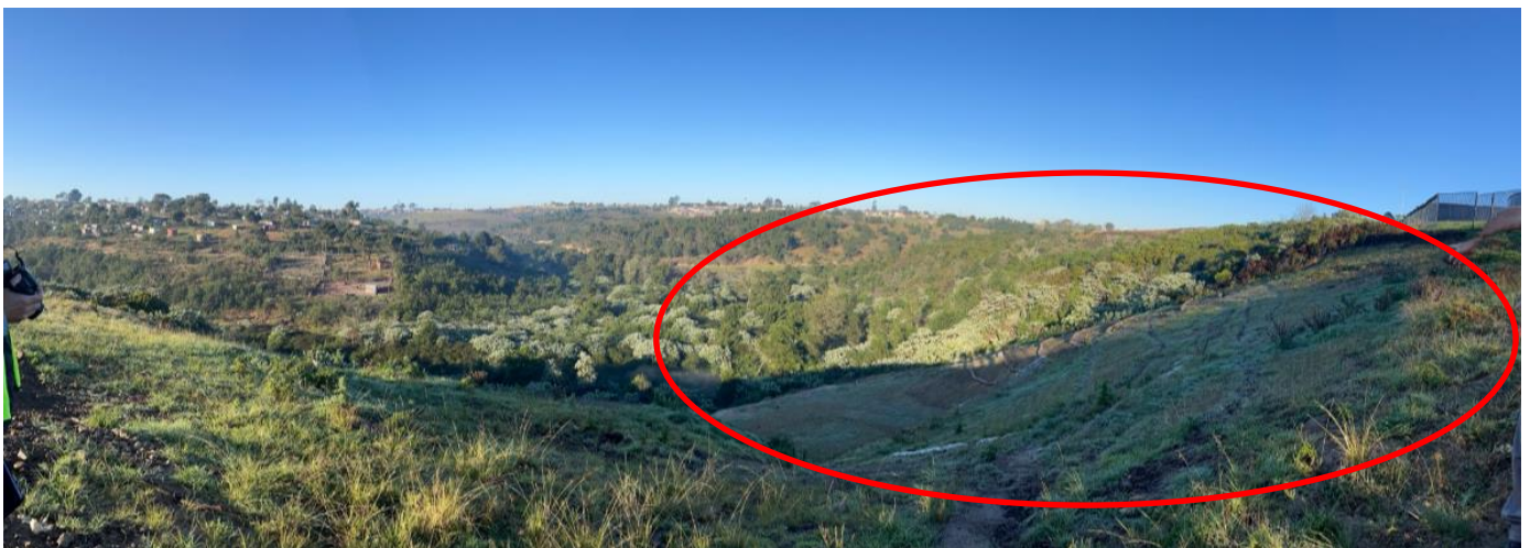
Figure 7: View of unlawful rehabilitation works undertaken at eroded area caused by the main stormwater outlet pipe (circled in red).
