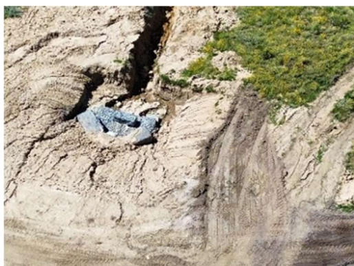
Temporary headwall and dissipator constructed at the stormwater outlet. Note there is still significant erosion below this structure and headward erosion will eventually result in the formation of a similar gully to the one that has just been the target of the rehabilitation effort (photo Zutari, November 2023)
