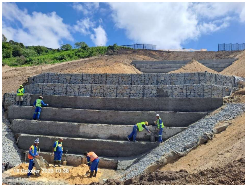
Gabions installed and donga being backfilled (photograph taken 18 October 2023) - works all beyond the 32m buffer from the edge of the watercourse.
