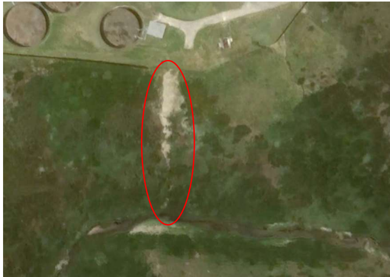
2022 Google Earth image showing the erosion gully/donga from the WWTW
