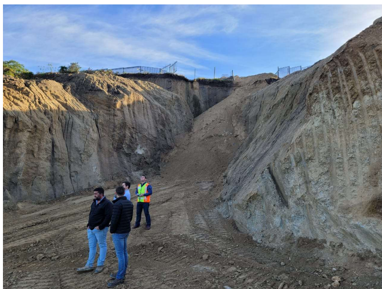
Donga/gully being filled and sloped to natural ground level (photograph taken July 2023)
