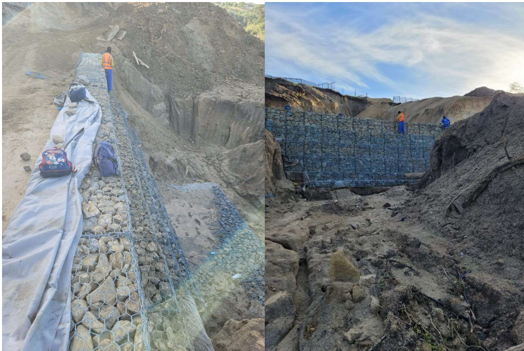
Retaining walls being installed to repair the existing donga (photograph taken July 2023)
