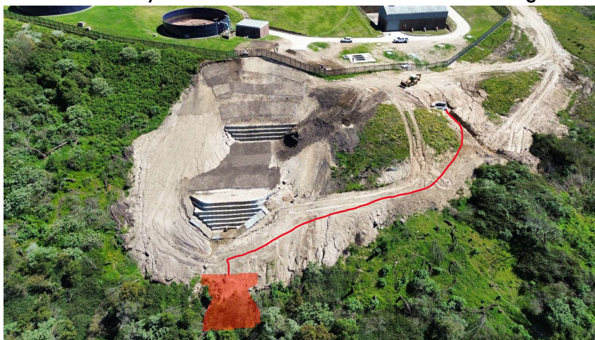
Drone photo showing the existing gabions installed (4m and 7m structures) and the approximate route of the new pipeline and outlet structure. Note that there has been no construction within the 32m buffer zone of the river, but that there has been overspill of material into this zone which needs to be rehabilitated.
