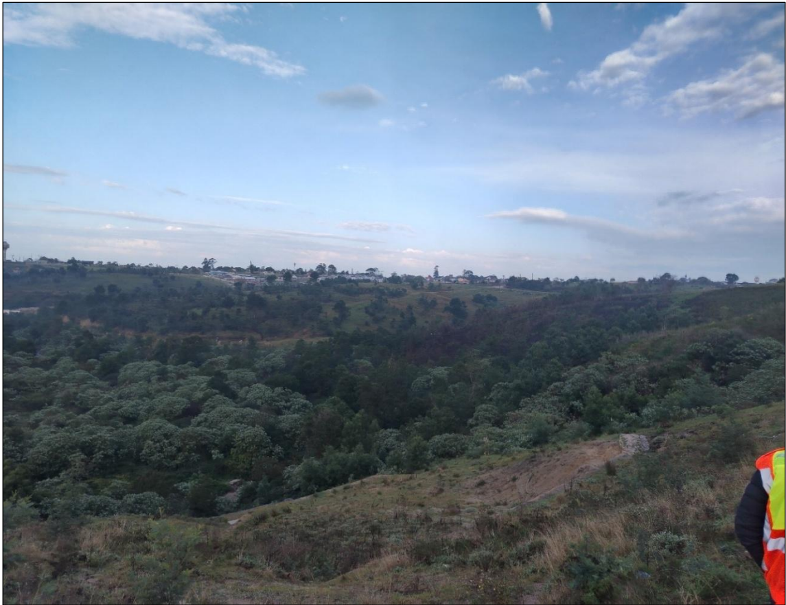
Image 3: Top angle of Rehabilitation work.
