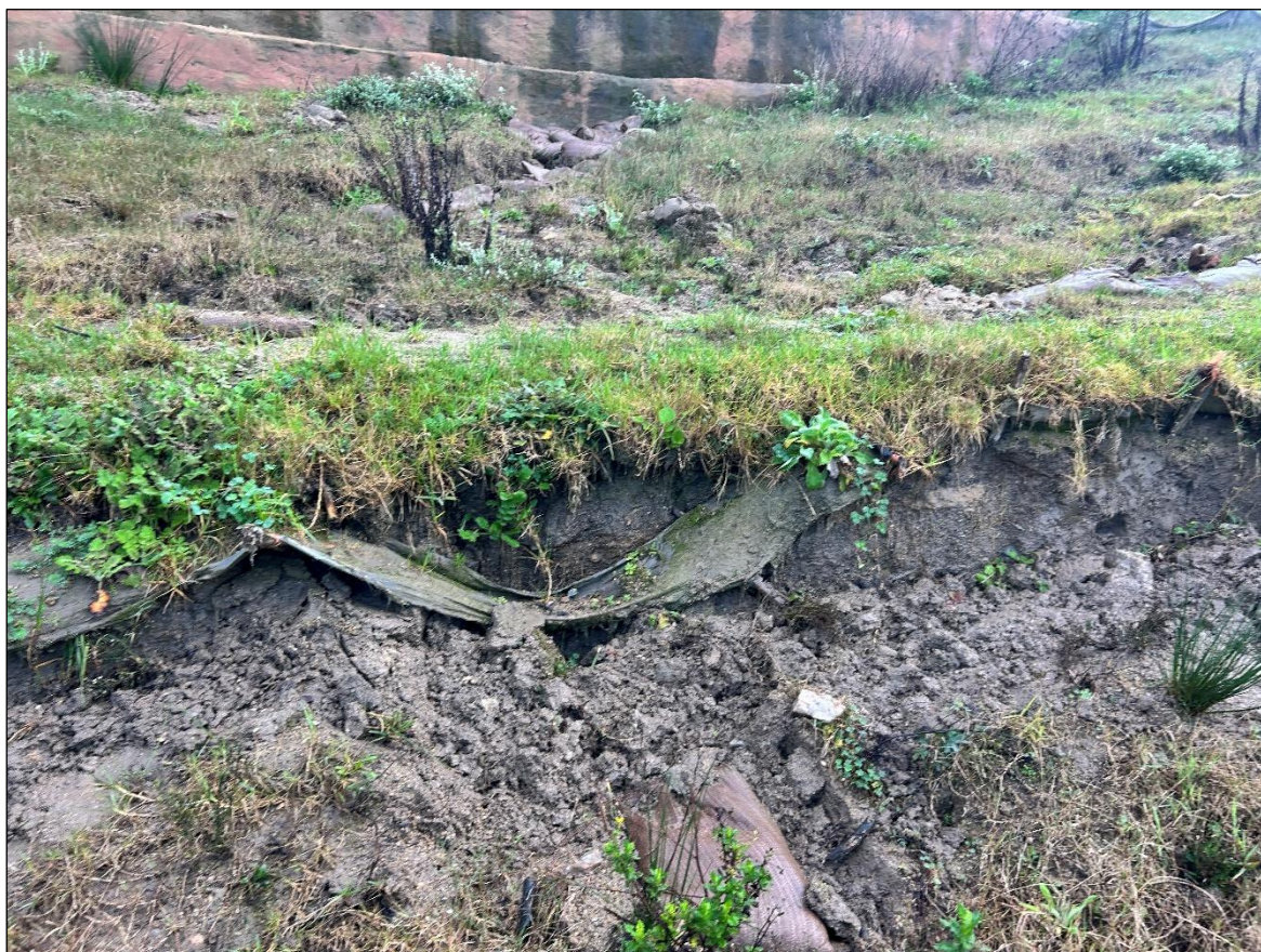
Image 8: Condition of the embankment stabilization measures (Geotextile Liner).
