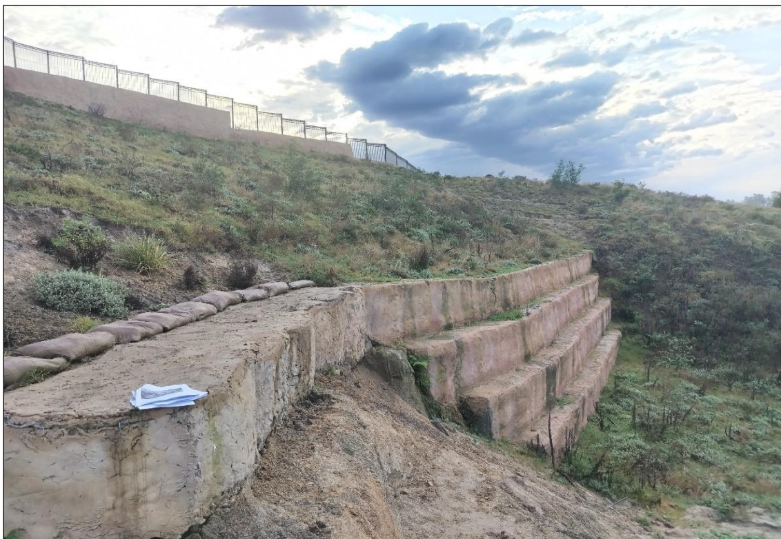
Image 2: Right Side angle of Rehabilitation work.
