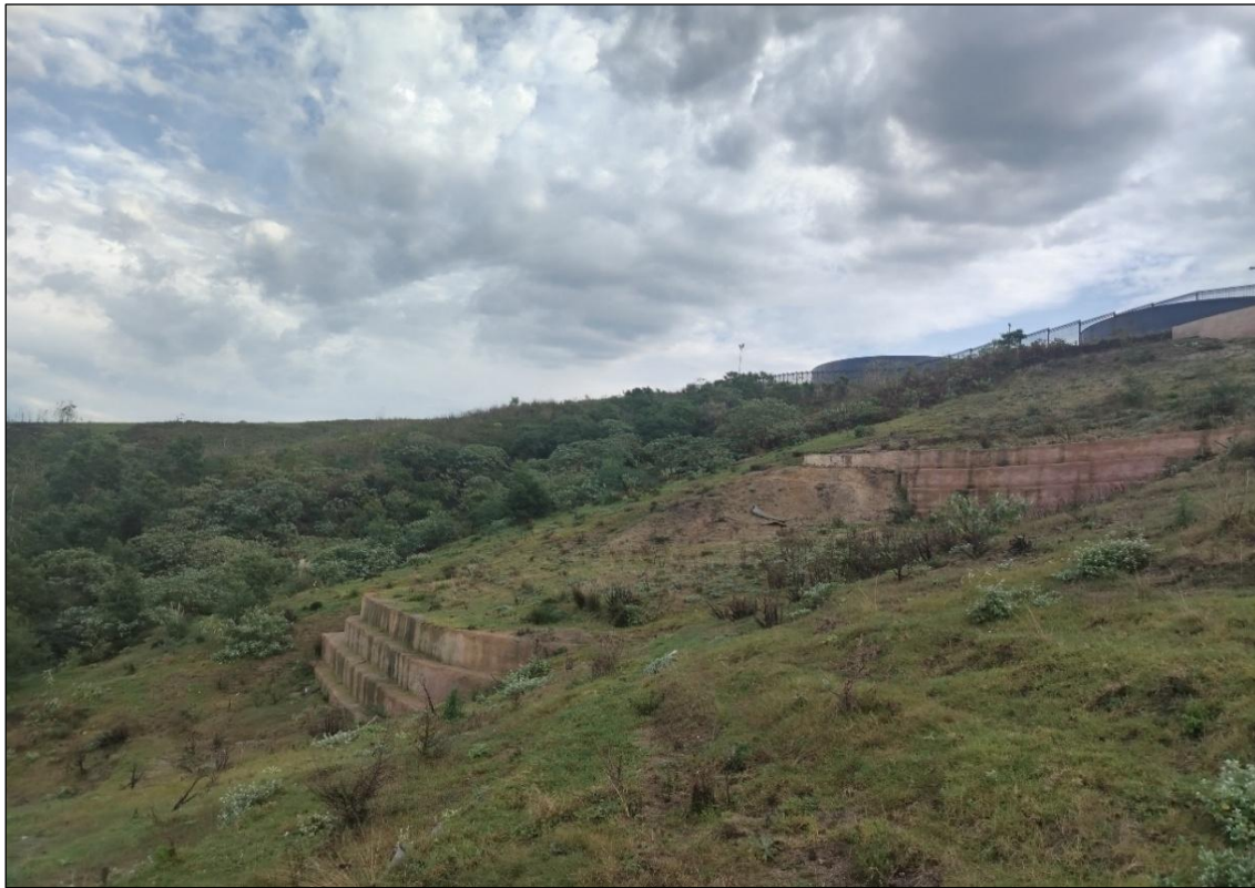
Image 1: Left Side angle of Rehabilitation work.
