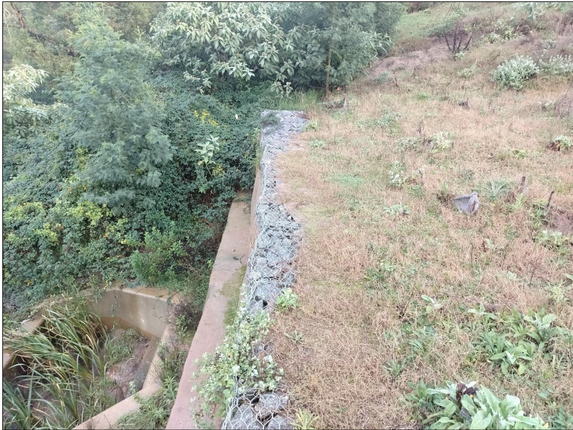
Image 5: Energy dissipating headwall.
