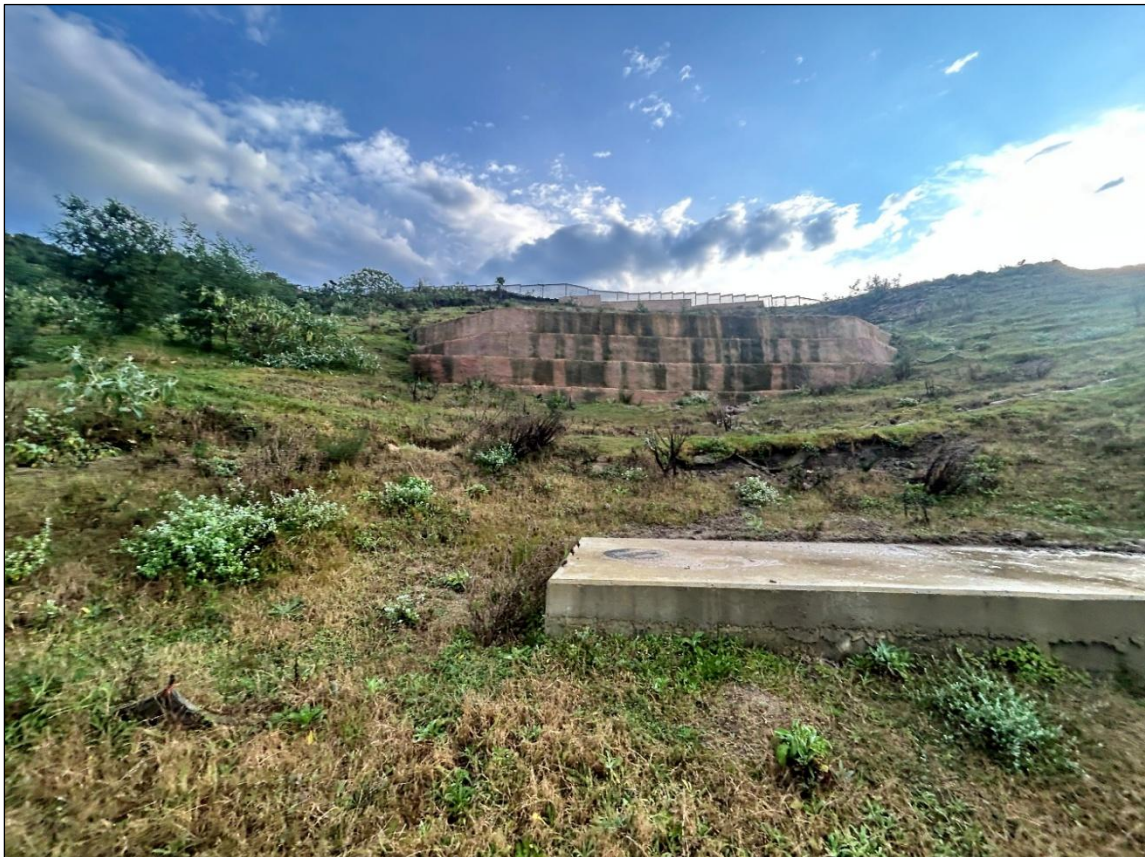
Image 4: Bottom angle of Rehabilitation work.
