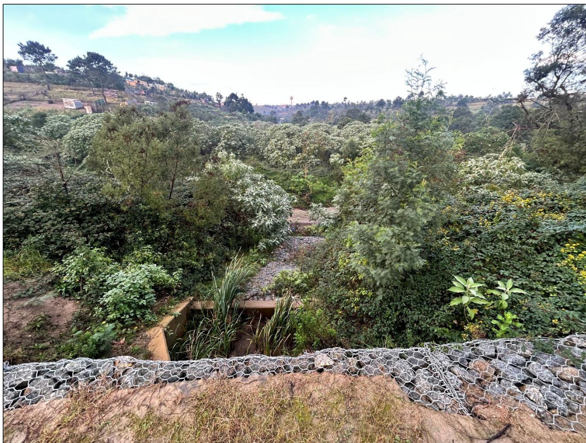
Image 7: Downstream view of the retention pond and associated gabion protection work.
