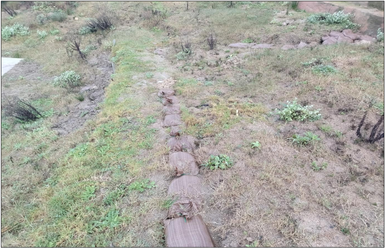
Image 11: Erosion control measures(Geotextile sandbags) implemented on the slope footprint
