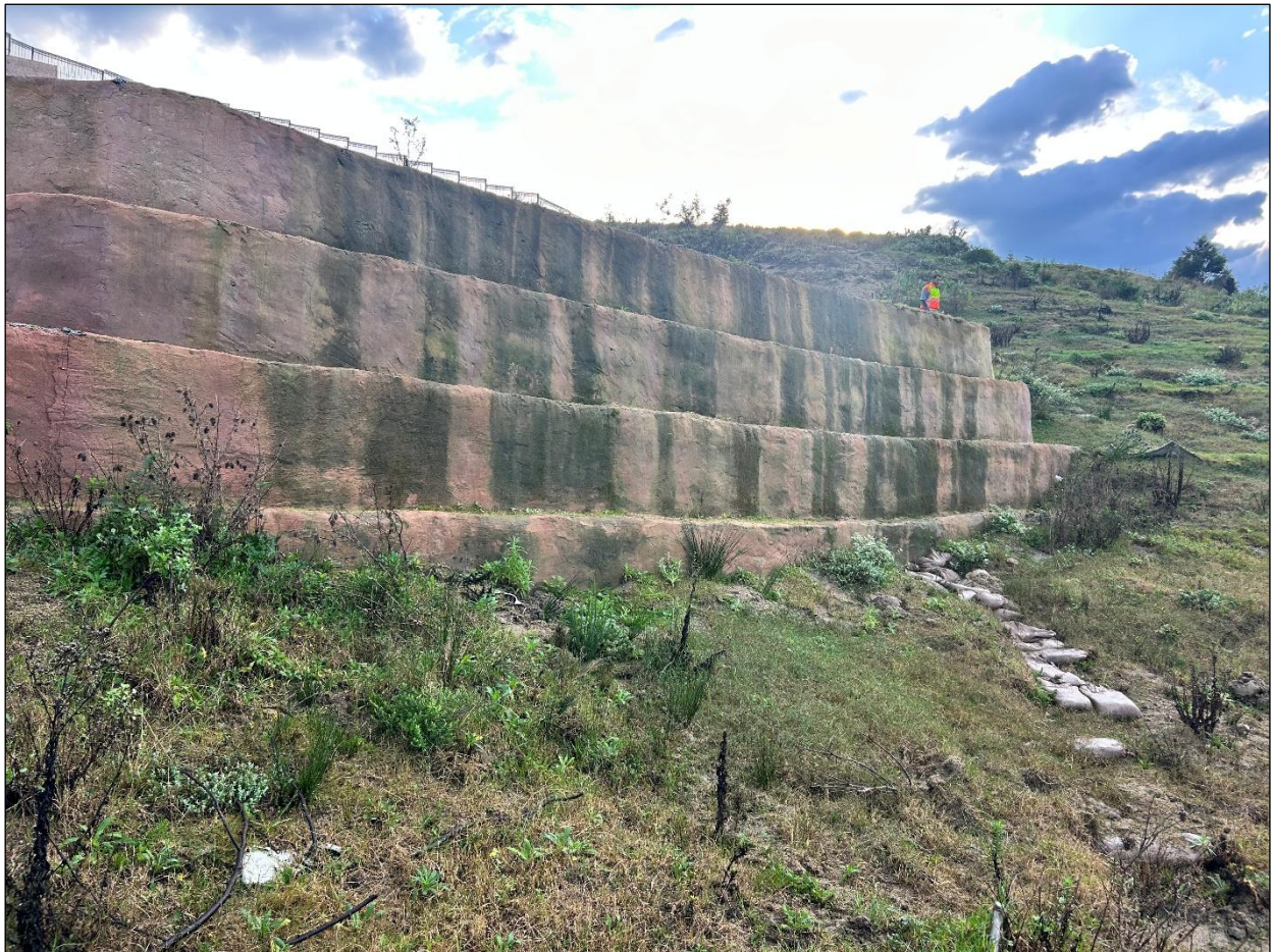
Image 10: View of the stepped retaining wall.
